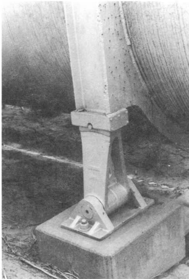
Photograph 6 - Rocker support and arm on the Malheur River Siphon - Owyhee Project.
