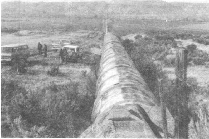
Photograph 2 - Bully Creek Siphon showing the riveted sections - Vale Project.
