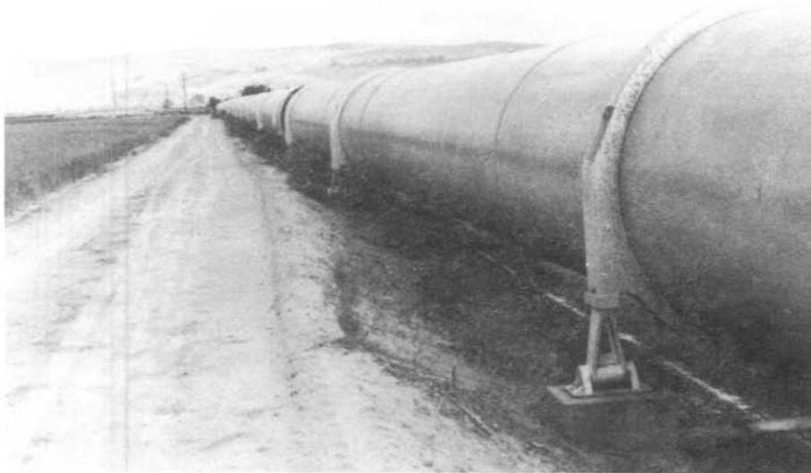
Photograph 1 - Malheur River Siphon showing the welded sections - Owyhee Project.
