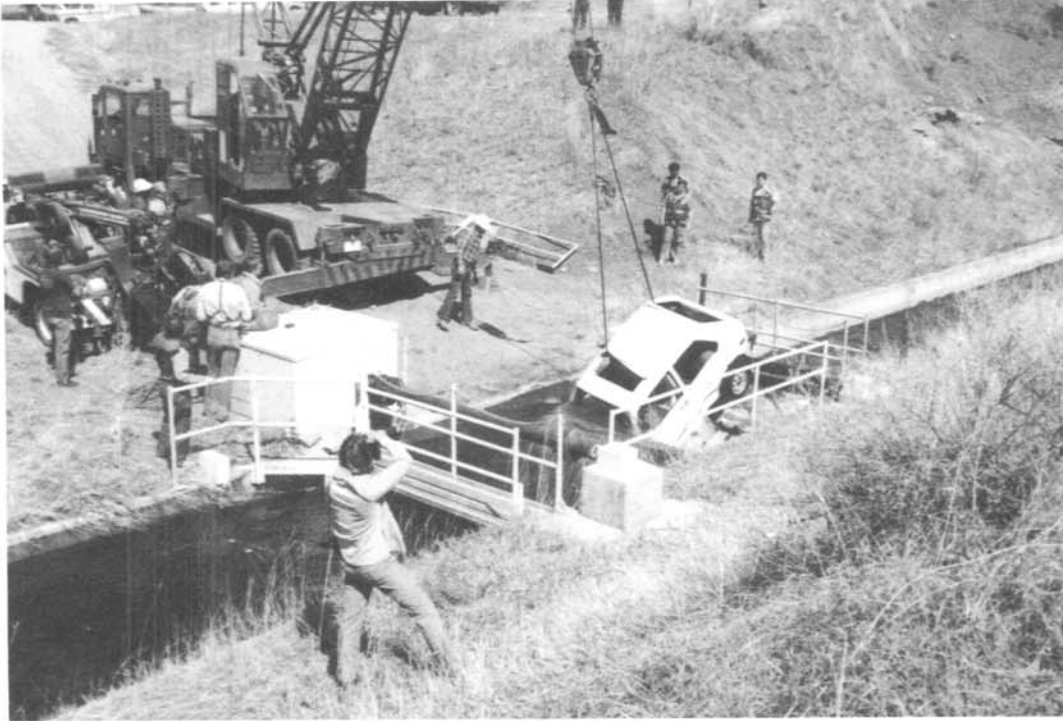
Photograph 4 - View of the trashrack structure, immediately downstream from a siphon. Fortunately, driver escaped from vehicle prior to passing through siphon. Colorado-Big Thompson Project.
