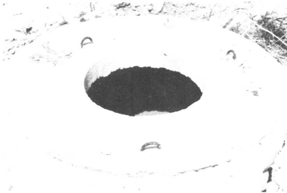
Photograph 21—Manhole cover deteriorating fast. Approximate age is 8 years old.
