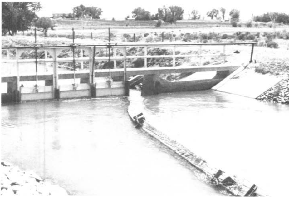
Photograph 19—Overflow spillway on check structure.
