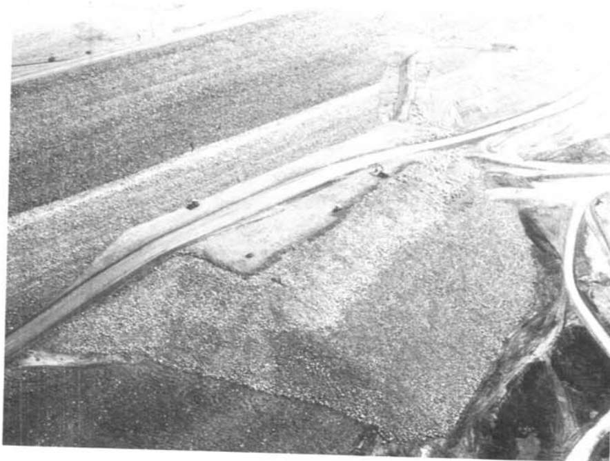
Construction of the stability berm.
