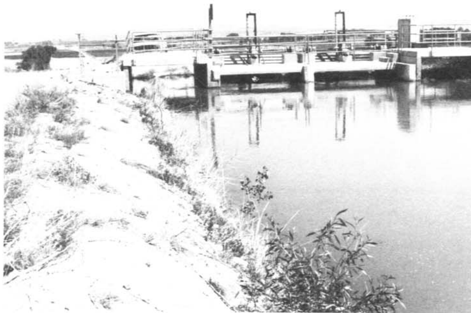
Photograph 2—Willows growing in membrane-lined ditch bank.
