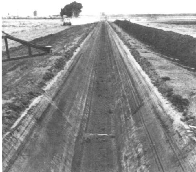
A new irrigation ditch.
