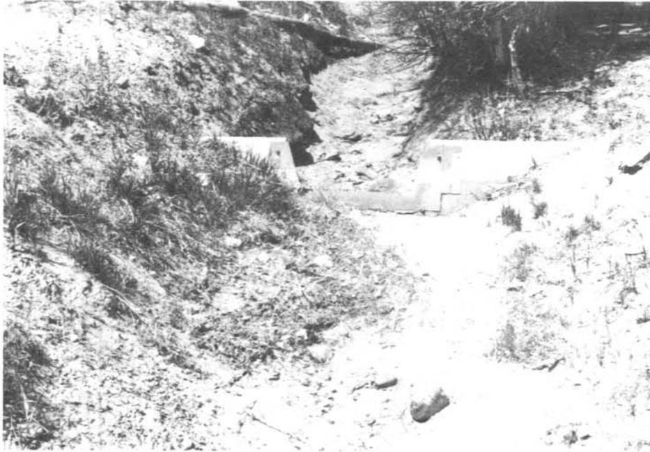
Photograph 13—Weir for making water flow measurements. Note silt accumulation in weir pool.
