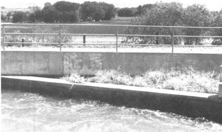
Photograph 18—Overflow spillway.
