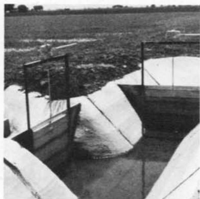
A newly constructed turnout structure on the Wellton Mohawk Irrigation District.
