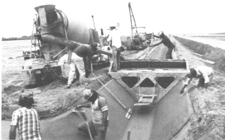
Pouring cement into a float, which forms the new irrigation ditch.
