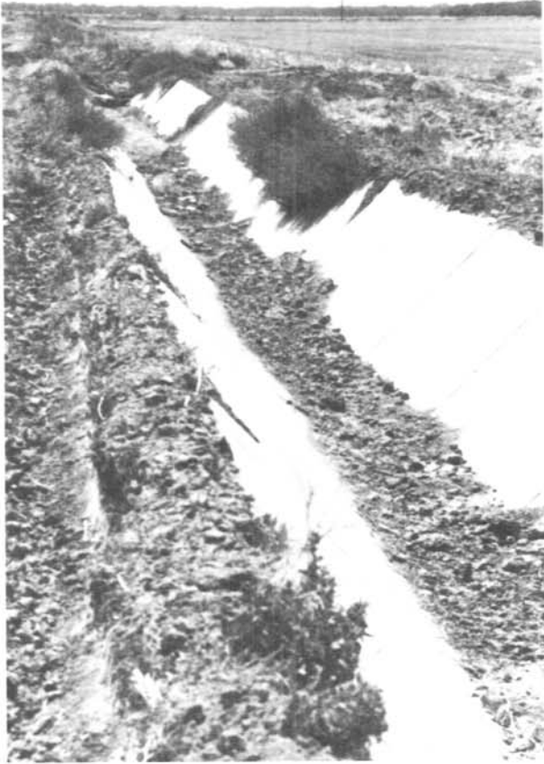
Examples of cracked, weed-filled irrigation ditches and gates.
