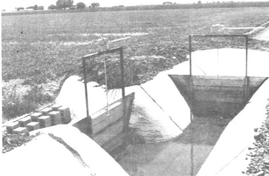
A newly completed turnout structure.
