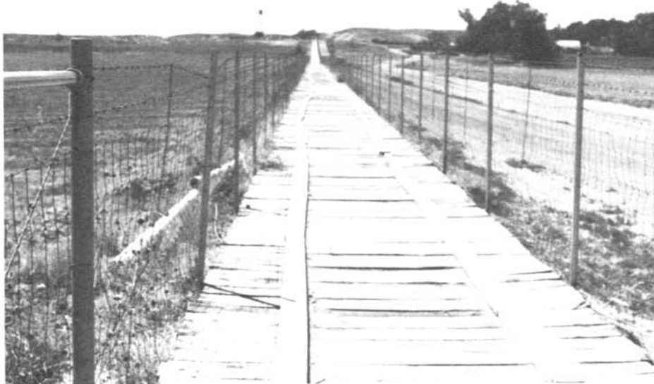
Photograph 9—The Pilot Canal Chute was covered with wooden members to control larvae activity. Uncovered portion is in background.
