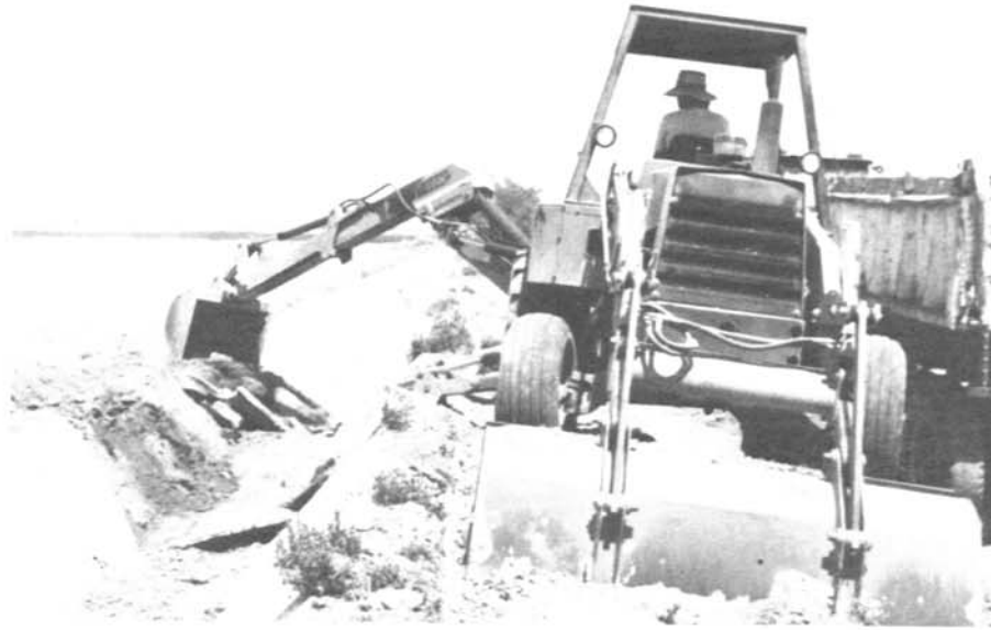
Ripping out an old ditch.
