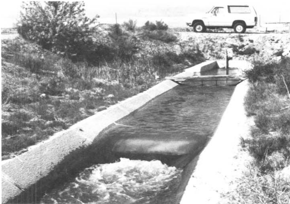
Photograph 10—Ramp flume and propeller meter (background).
