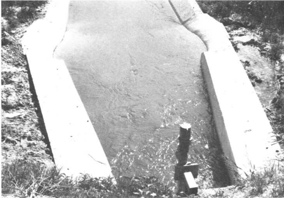
Photograph 11—Closeup of propeller meter.
