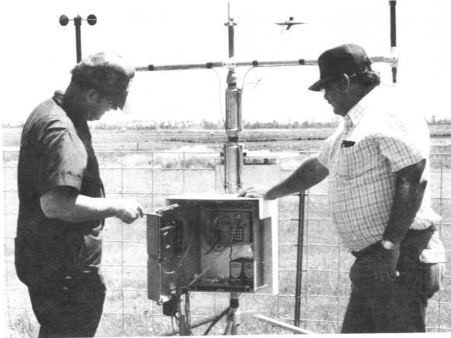
Extension agricultural engineers Delbert Schwab, left, and Sam Harp, examine a remote weather recording station used in irrigation scheduling.
