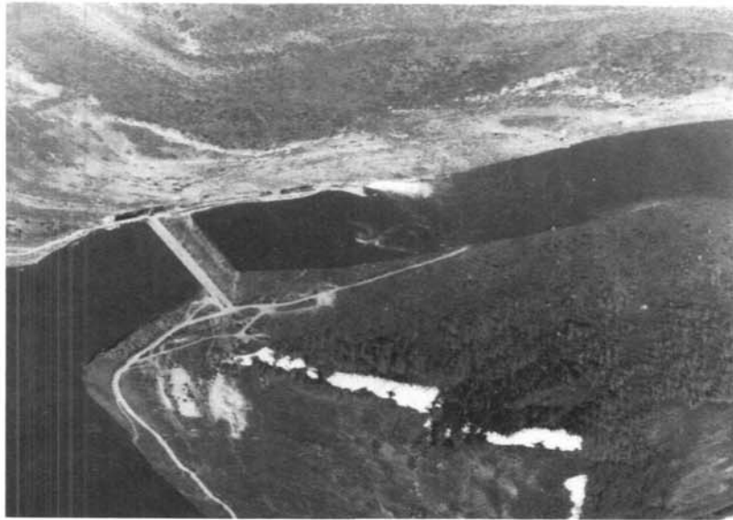
Aerial view of Strawberry Dam looking southwest. Soldier Creek Reservoir is to the left of Strawberry Dam in this photograph.
