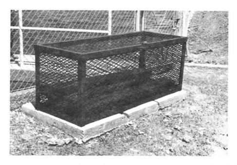
Since installation of the stoplog box shown in the photographs, very little loss and vandalism have been experienced on the box itself and the stoplogs.
