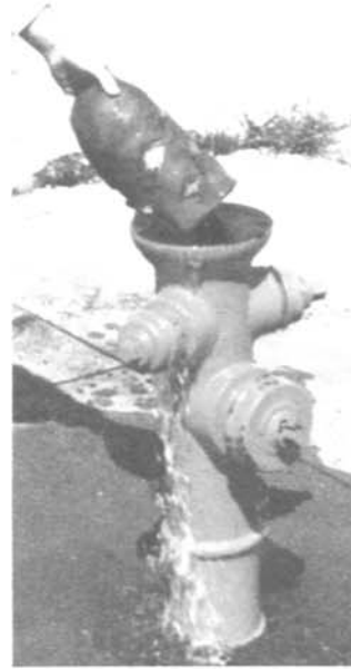
Pig being recovered from a fire hydrant.
