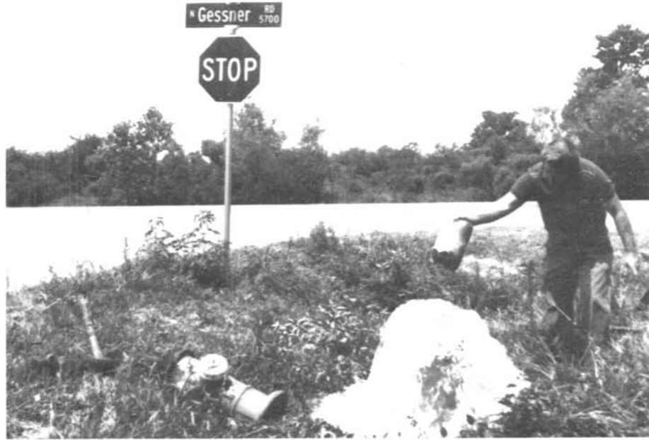
Above, flushing the line after pigging.
