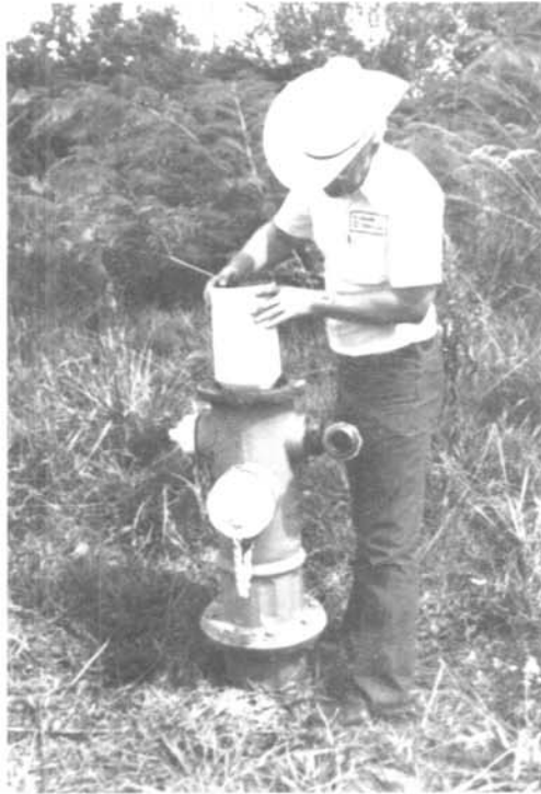
Pig being launched into a fire hydrant.
