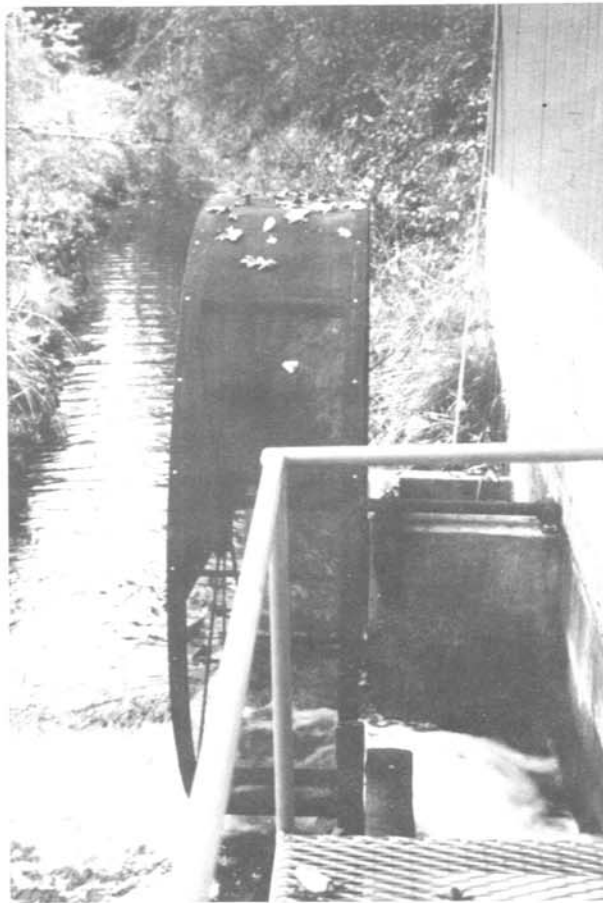
A simple turn gate, located at the bottom of the upper photo, directs water from the upper canal into the pipe which feeds the Reed Road generation unit. The water (lower photo) then flows from the turbine into the lower canal.
