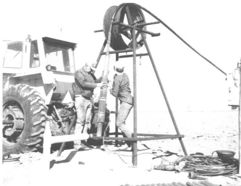
Lowering tubing Into a well
