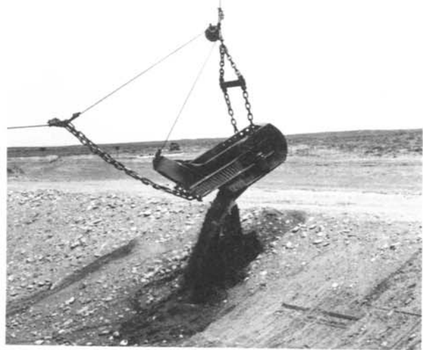
Figure 5.—Placement of protective earth cover.
