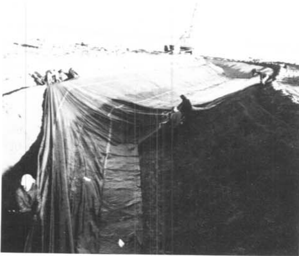
Figure 4.—Installation of membrane.
