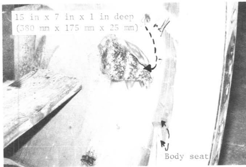
Figure 4. Cavitation damage to hollow-jet valve body.
