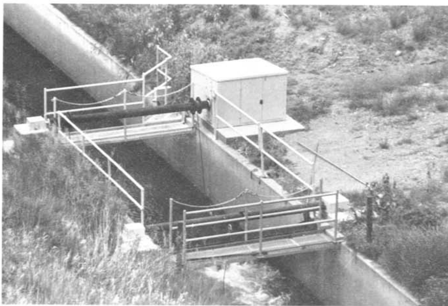
Figure 2.—Downstream view of structure showing the pivoting trashrack, walkways, and railing.
