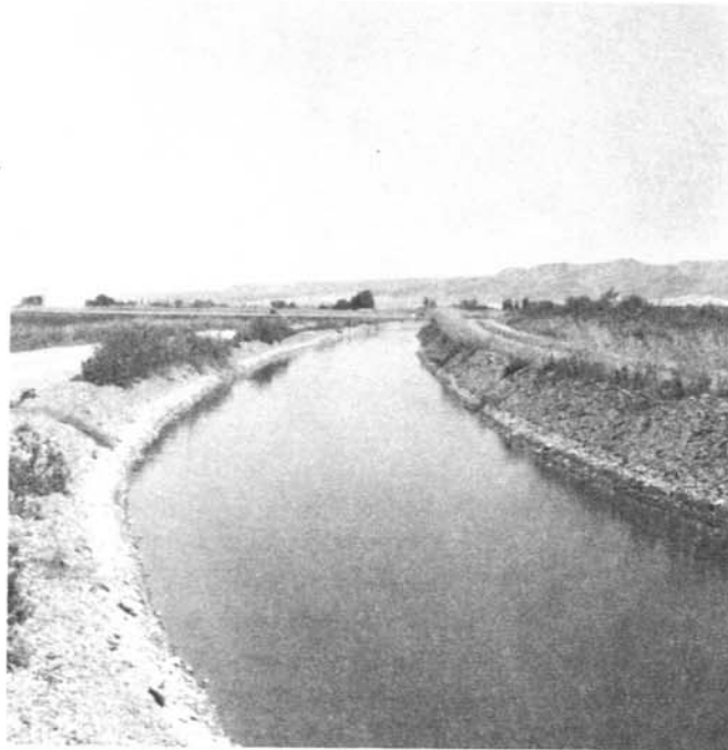
Figure 3.—"G" canal in the second year of operation after lining work.
