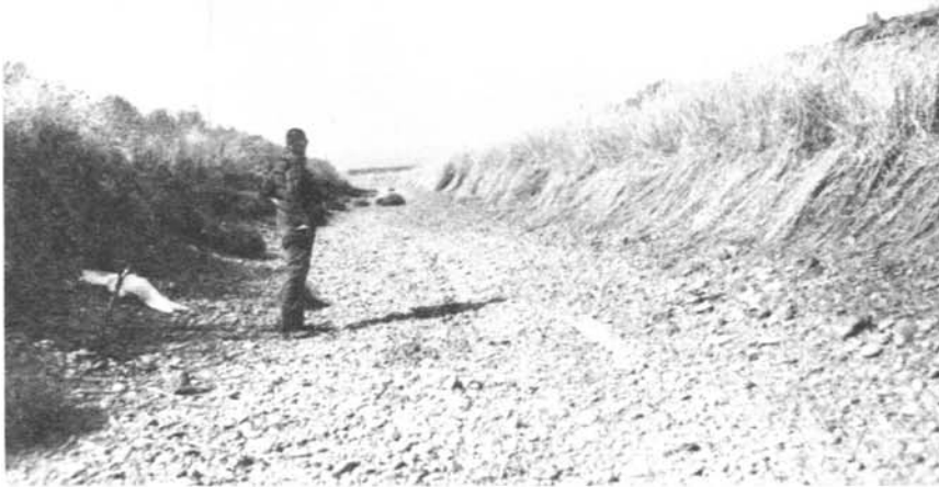
Figure 10.—Granular cover on Kennewick Main Canal.
