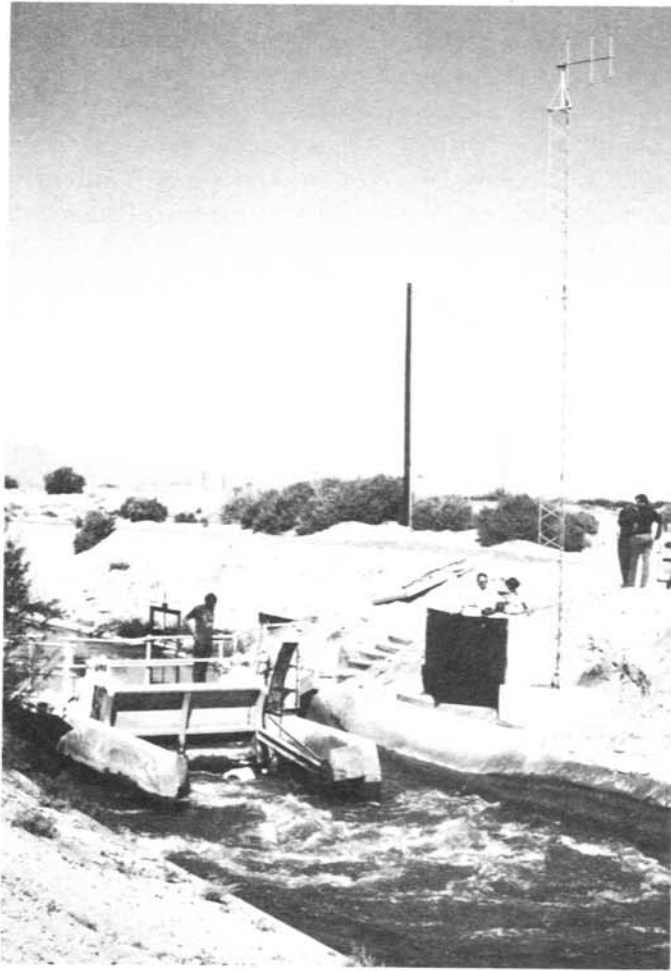
Figure 5.—Check structure rehabilitation and control equipment installation.
