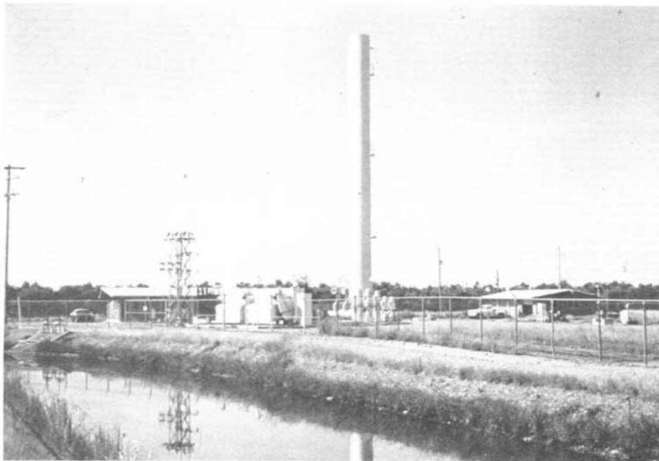
Figure 13.—Automated canalside pumping plant.
