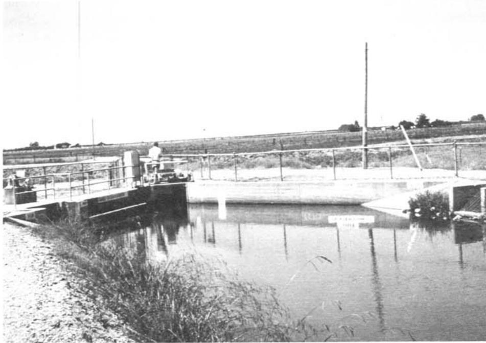
Figure 9.—Radial gate check structure.
