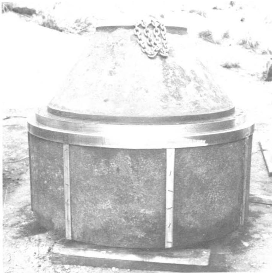
Figure 17.—Body extension after overhaul—54-inch interior differential needle valve.
