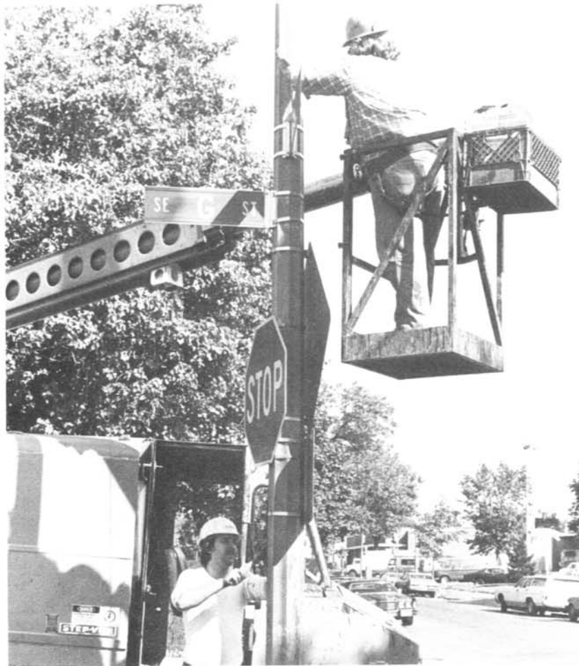
Figure 1.—Wire brushing street light pole.
