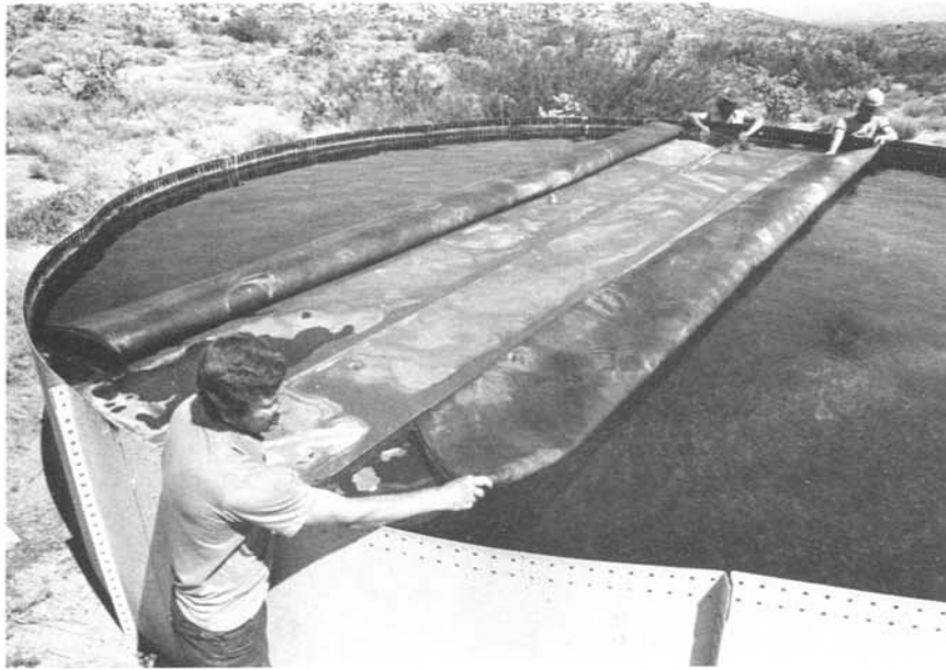
Figure 9.—The cover is being unfolded onto the water's surface. Puncture holes in the cover allow rain water to enter the tank and prevent the cover from sinking. This particular water tank has holes around its rim allowing excess water to leak out.
