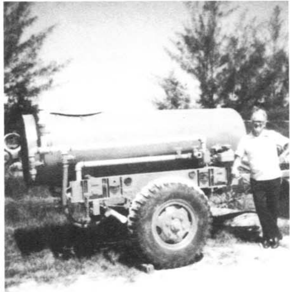
Figure 5.—Water trailer for maintenance jobs.
