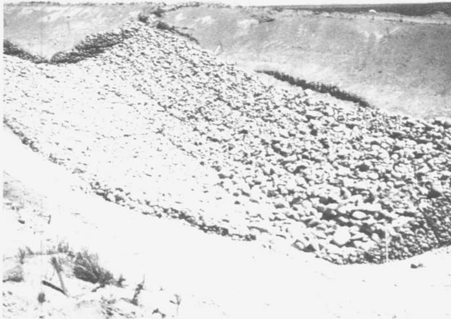
Figure 1.—Completed gabion drop with gabion control notches.
