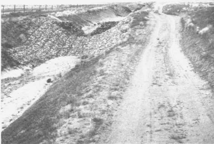
Figure 6.—Gabion drops installed in block 2.
