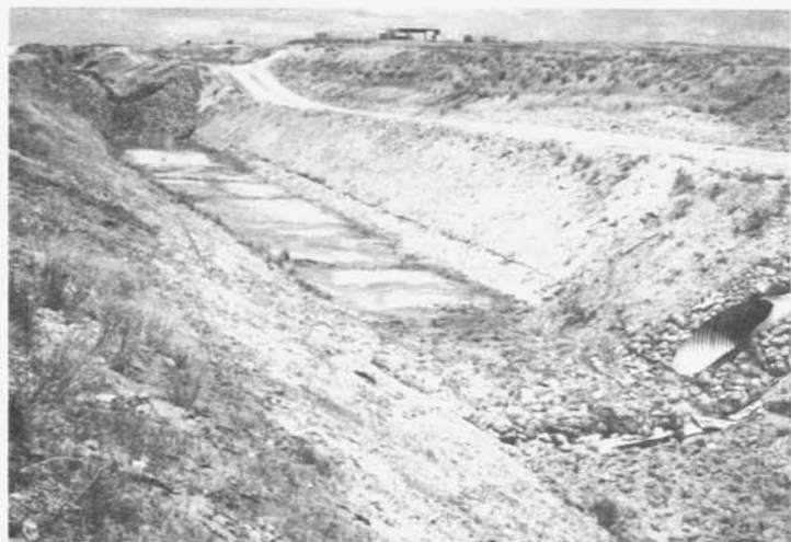
Figure 5.—Gabion riprapped inlet structure on collector drains underlain with filter cloth.
