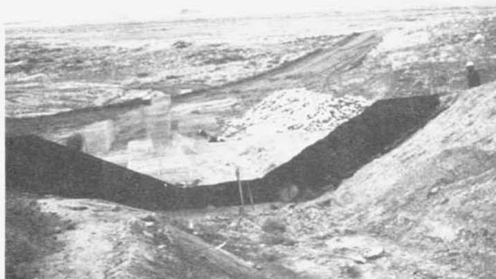
Figure 7.—Gabion drops currently under construction in block 3.
