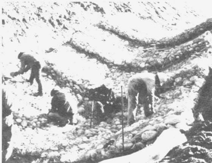
Figure 3.—Placing preselected and sorted rocks in gabions.
