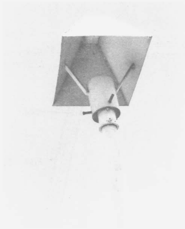
Figure 4.—Protective device for light bulbs.
