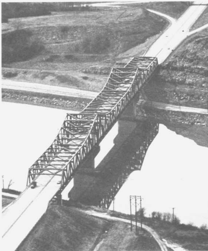
Figure 18. Bridge carrying Interstate 64 across the Kanawha River.
