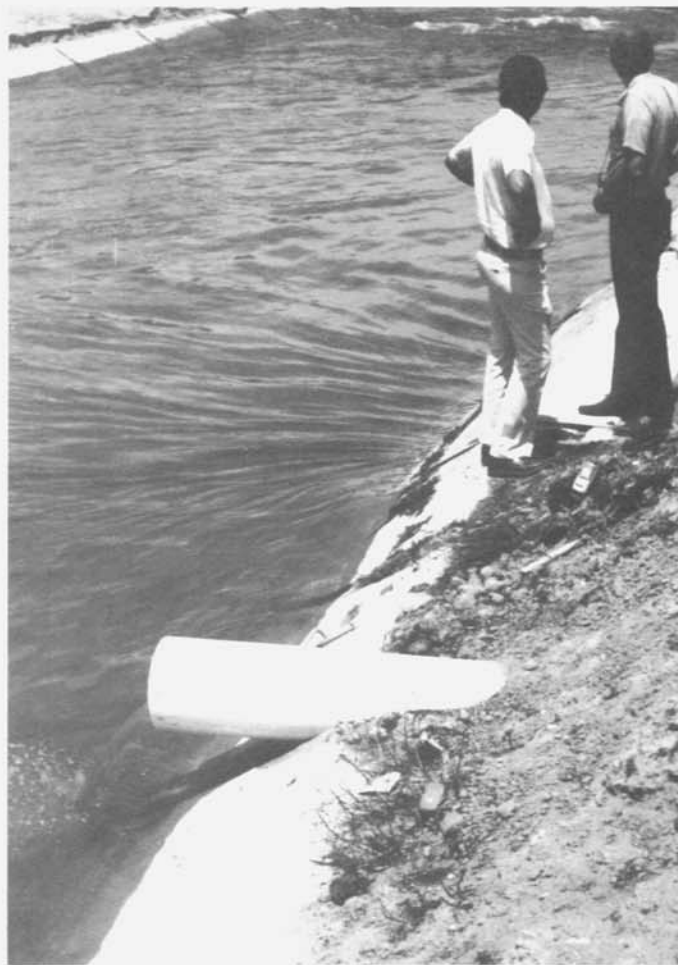
Figure 10. PVC drainpipe returning wash water and moss to main canal.
