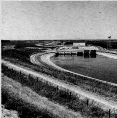
San Luis Unit, Water and Power Resources Service's Central Valley Project, California. Shown in the picture is the Dos Amigos Pumping Plant and San Luis Canal near Los Banos, California. This plant contains six pumping units that lift water 38 m (125 ft) to reach 2 of the San Luis Canal. From that point on, gravity pulls the water southward.
