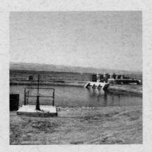
View of pumping plant 7R-B, a regulating reservoir that controls the pumps at pump lateral 7R-A, a few kilometers west of Tranquility, California. This is one of three reservoirs needed to pump and deliver water on the uphill side of the San Luis Canal. It is part of the Westlands Water District distribution and drainage system being constructed by the Water and Power Resources Service as part of the San Luis Unit, Central Valley Project.
