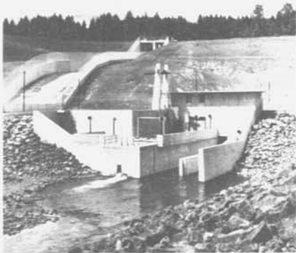
Scoggins Dam outlet works control house and fish handling structure, Tualatin Project. The spillway and top of the dam are visible on the left.
