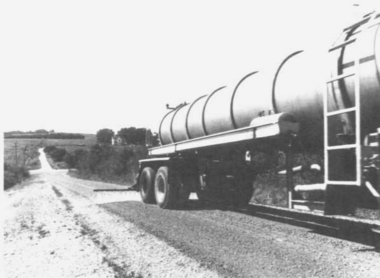
Figure 2.—Tanker above shows a typical method for applying calcium chloride to crushed rock roads.
