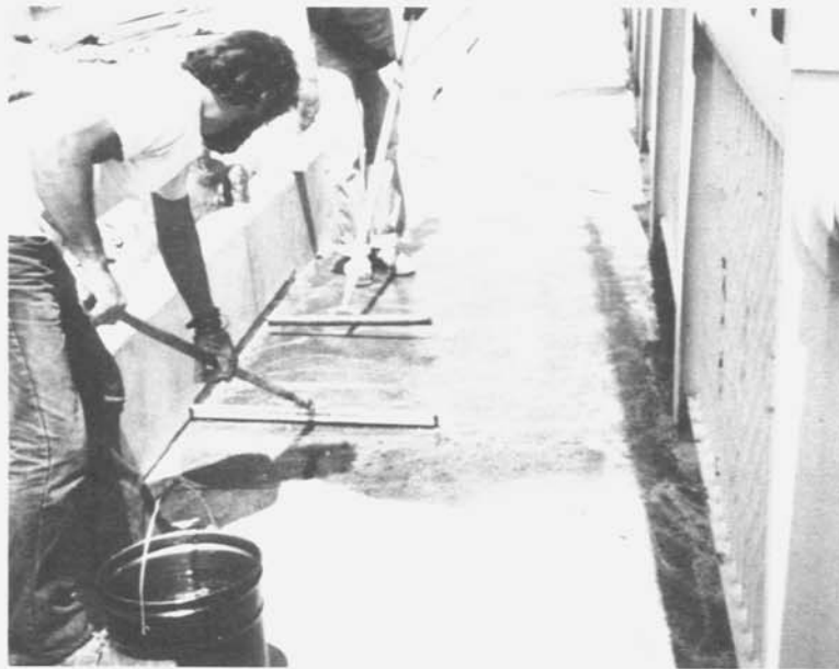
Figure 8.—Protective coating of epoxy material is squeegeed on bridged walkway.
