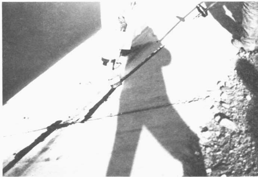
Figure 4.—Applying rubberized asphalt.
