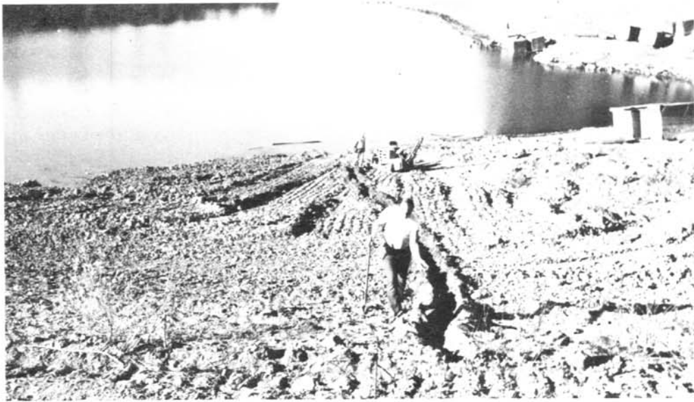
Figure 3.—Anodes placed along the reservoir shore were connected by a single buried cable to the 30-V rectifier.
