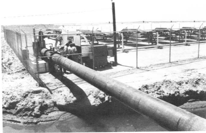
Figure 4. - Tailwater pumped into the irrigation ditch is delivered via this metallic pipe connecting the ditch with the solar pump.
