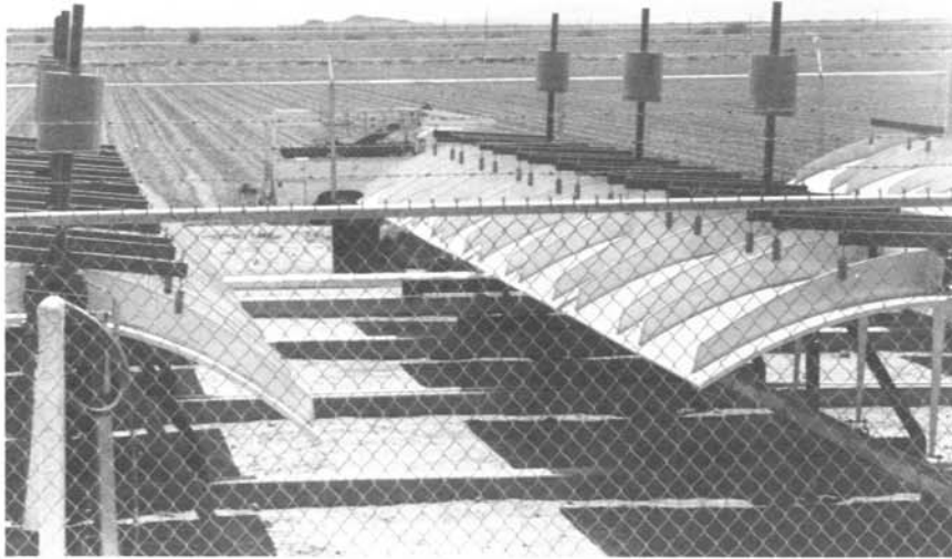
Figure 5. - The solar concentrators shown in a "stowed" position. During hours of calm weather and daylight, the collectors are faced upward where they track the sun across the sky.
