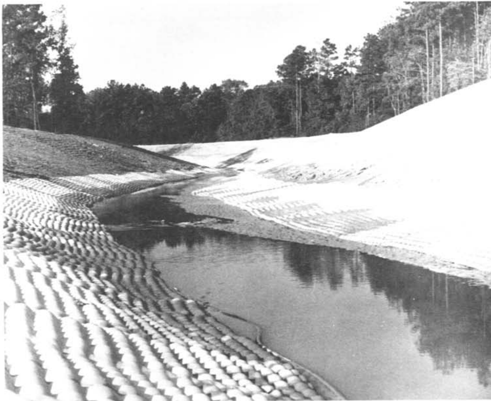
Figure 1. - Sand and silt that settle in the low pockets of the Fabriform mat can support vegetation growth. The cobblestone effect is caused by the spot woven filter points in the mat.
