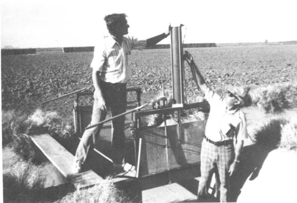
Figure 1. - This photograph shows a jack-gate that has been automated in an irrigation system near Yuma. Air entering the bottom of the cylinder opens the gate while air entering the top of the cylinder closes the gate. Eight such gates irrigate 26.30 hectares (65 acres) in this plot - four gates to a "set."
