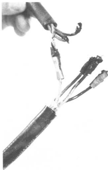
Frayed wiring, such as this piece removed from a center pivot, caused death of a Wyoming man this year.
