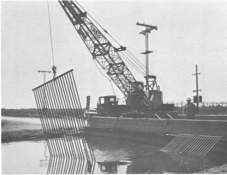
Figure 13. Dragline shown placing grates in canal. Photo PX-D-60889.
