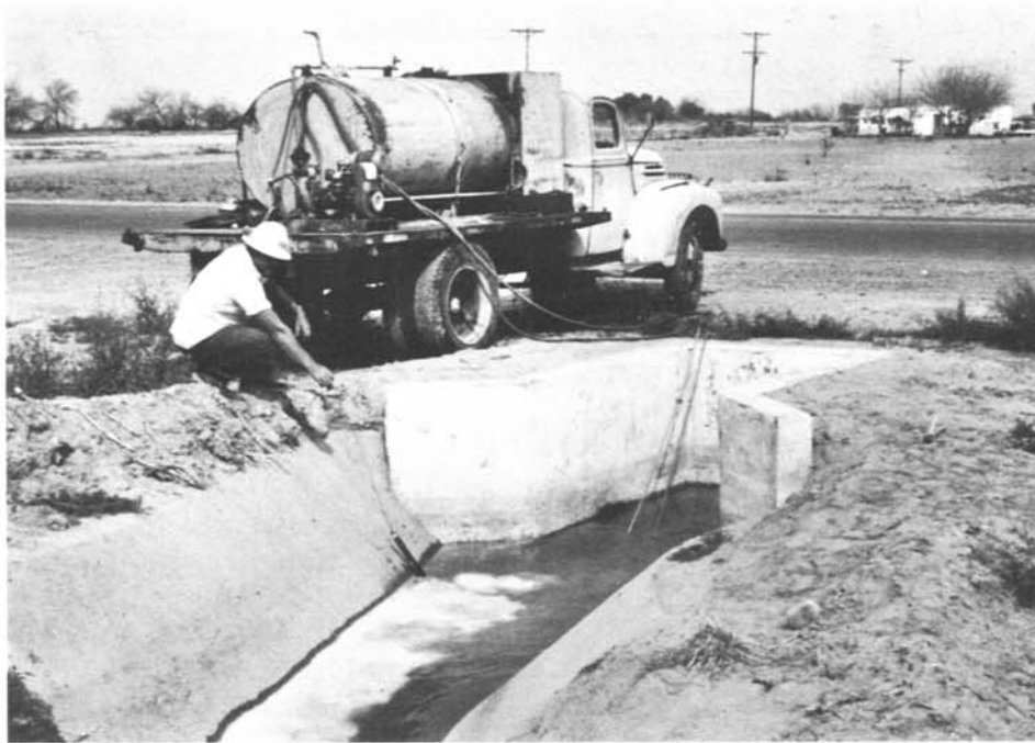
Figure 19. Solvent being introduced into a pump and drainage channel. Photo PX-D-60894.
