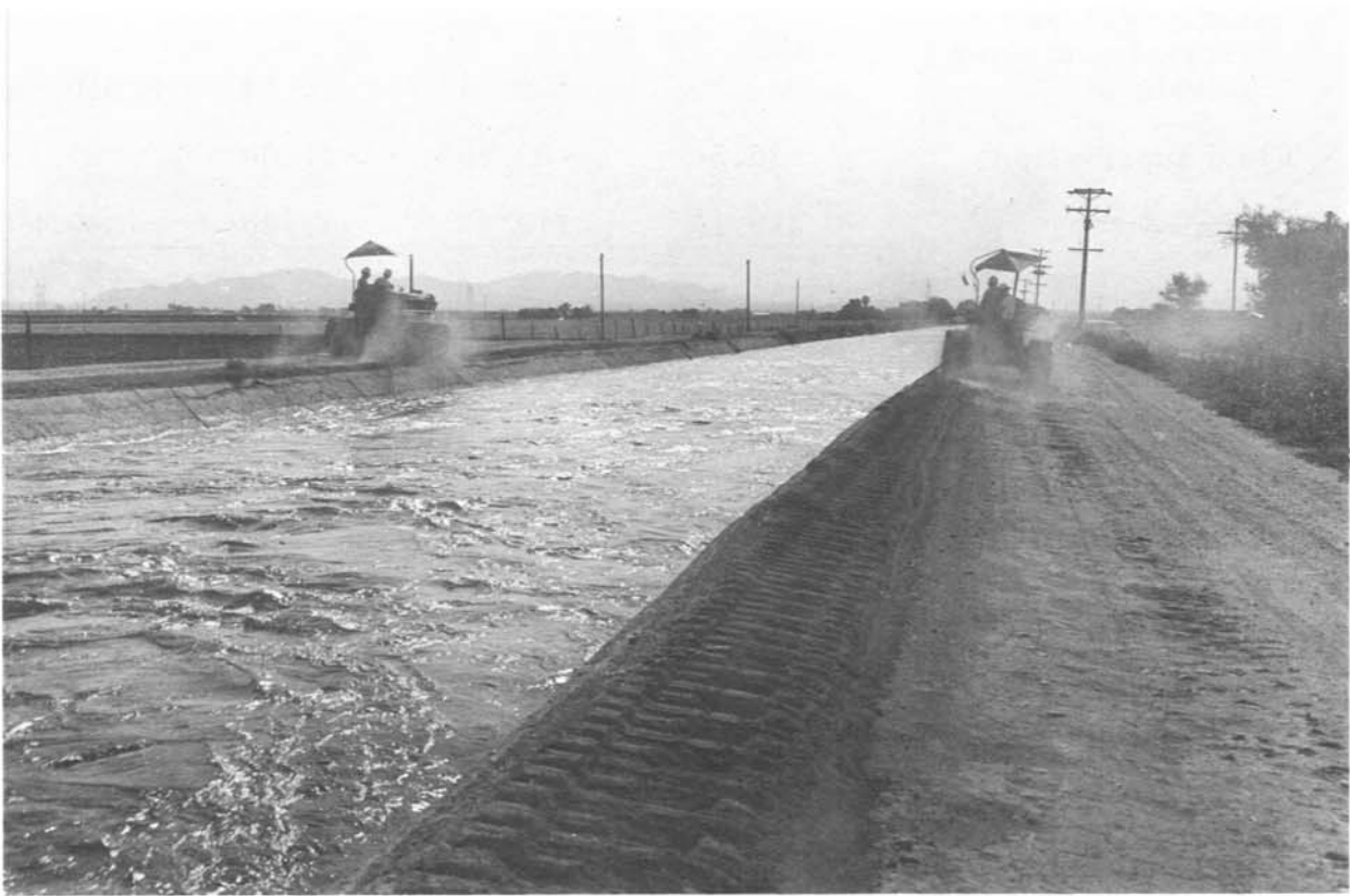
Figure 10. Dislodging aquatic weeds and silt by the anchor chain and disc method in the Grand Canal. The chains and discs in the canal are not visible. Photo PX-D-60886.
