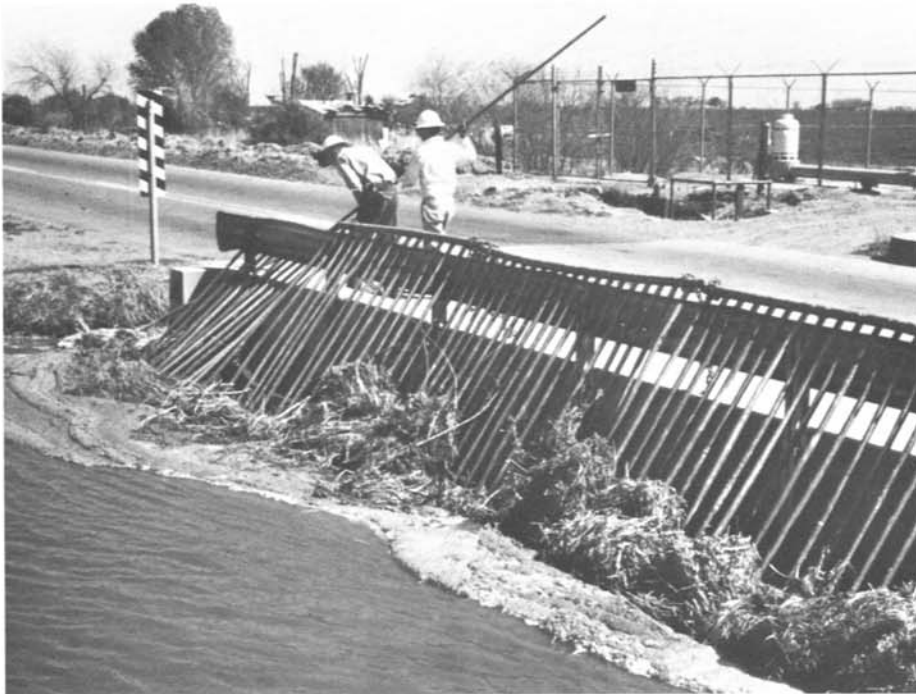
Figure 14. Removal of aquatic weeds from grates. Photo PX-D-60890.
