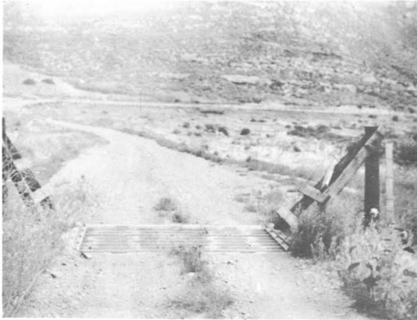
Photo 5 - A typical cattleguard of standard design but with reduced dimensions, installed on the Colorado-Big Thompson Project.
