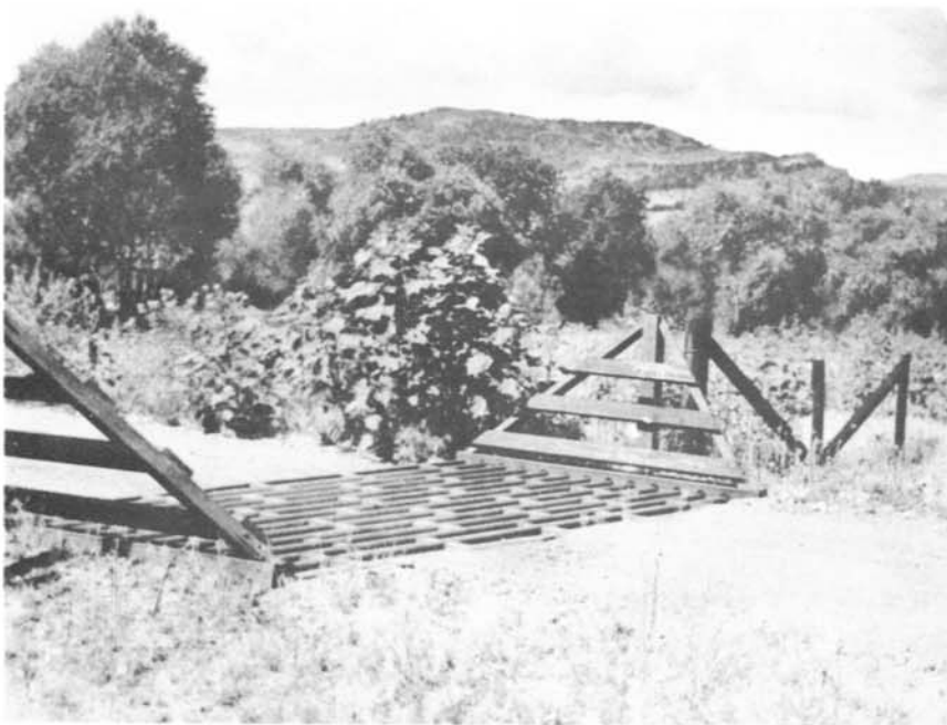
Photo 6 - A typical cattleguard of standard design and full dimensions, installed on the Colorado-Big Thompson Project.
