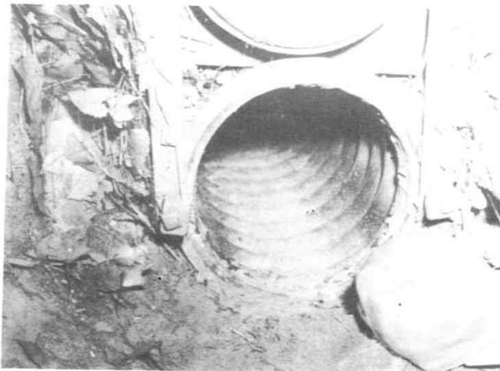
Photo No. 10 Fountain Mutual Irrig. Dist.
