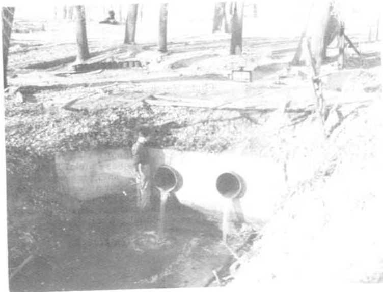
Photo No. 11 Fountain Mutual Irrig. Dist.
