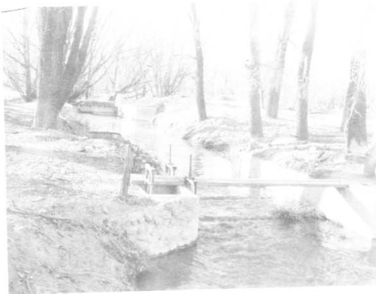
Photo No. 12 Fountain Mutual Irrig. Dist.
