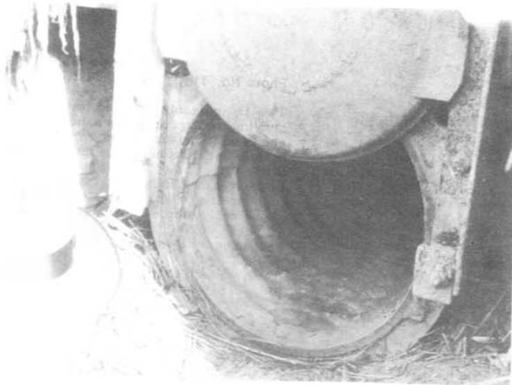
Photo No. 8 Brantner Extension Ditch
