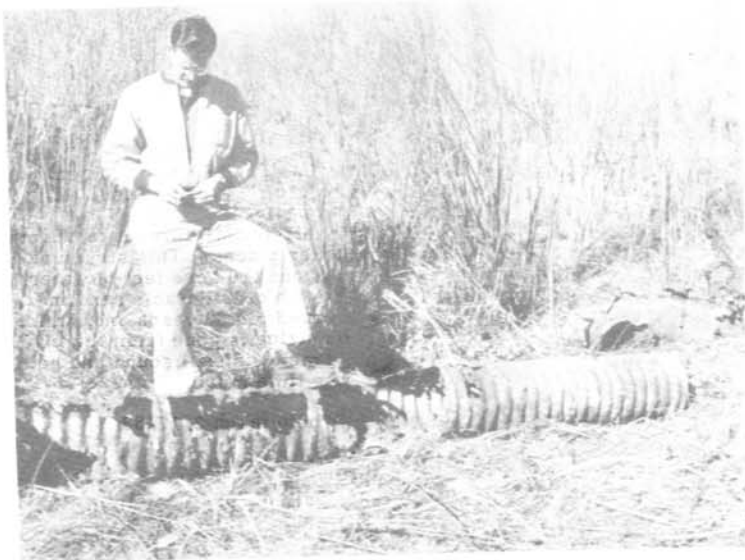
Photo No. 13 Fountain Mutual Irrig. Dist.
