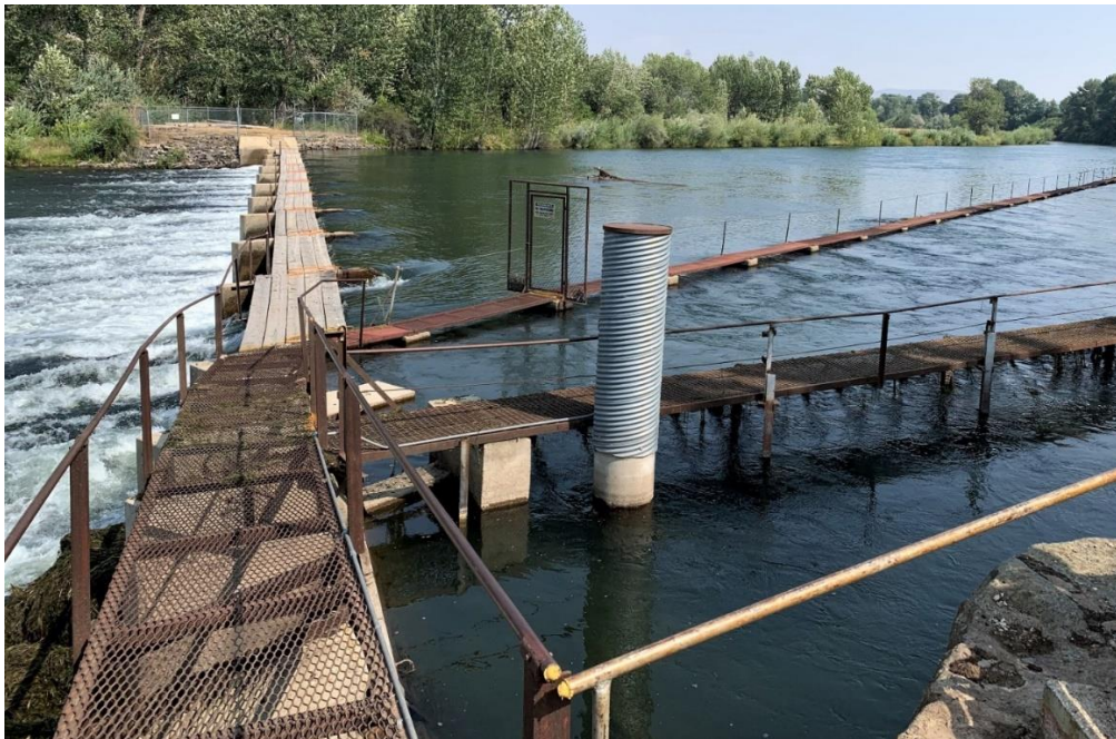
Figure 2 Existing Ridenbaugh Diversion Structure
