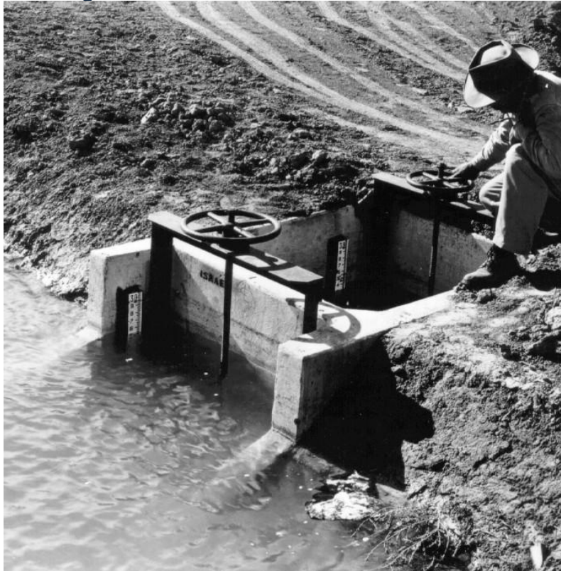
Figure 3 – Head Differential Measurement
