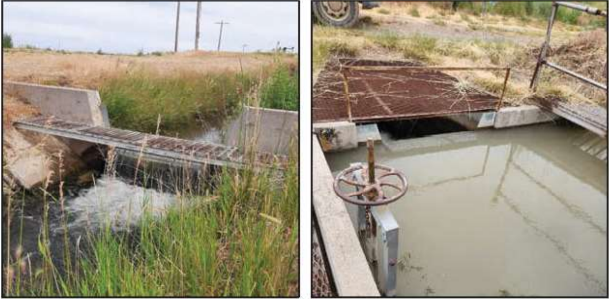
Figure 6 Spillways on East (left) and West (right) canals
