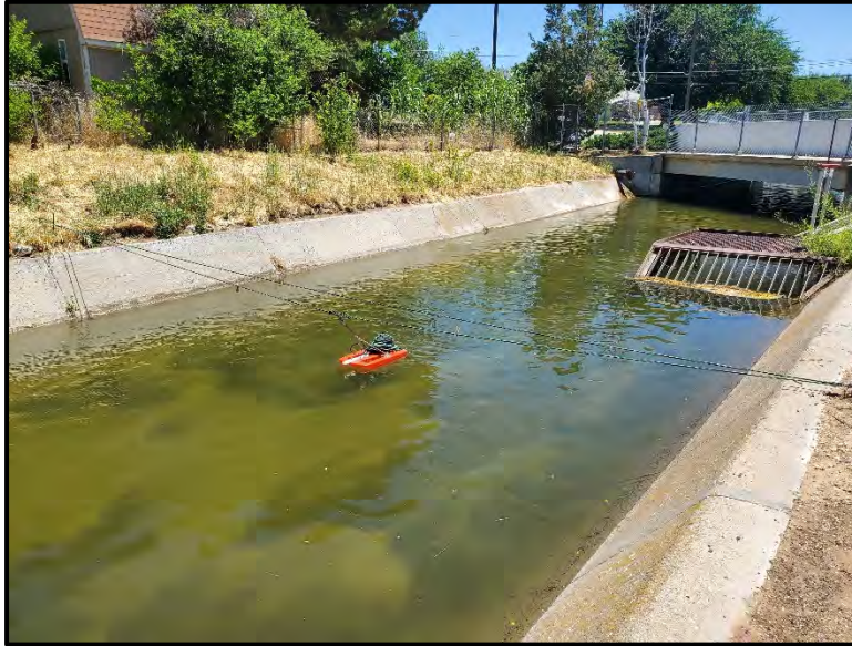
Figure 2 - ADCP flow meter at 300 North, downstream location of Segment 38
