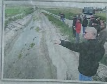
Alan Rollo of the Sun River Watershed Group, talks about how lining a canal in the Fort Shaw Irrigation District has saved water.
