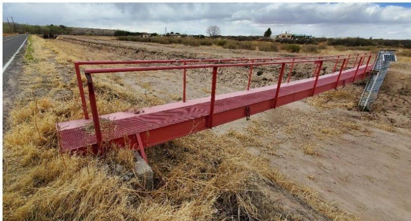
*Figure 5. Photo of existing metering bridge looking upstream*
