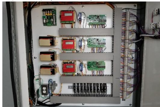
*Figure 3. EBID SCADA electronic controls of the "Electric Wasteway" of the Leasburg Main Canal*
