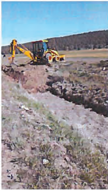
Figure 1. Downstream dam on Yonna Canal for HID ponding test.
