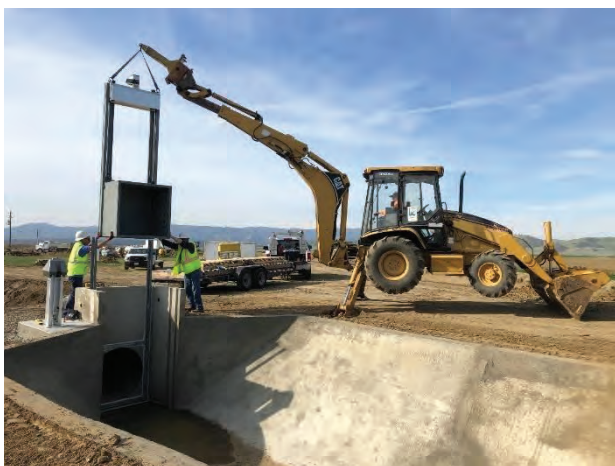
Fig. 6: Installation of SlipMeter gate
