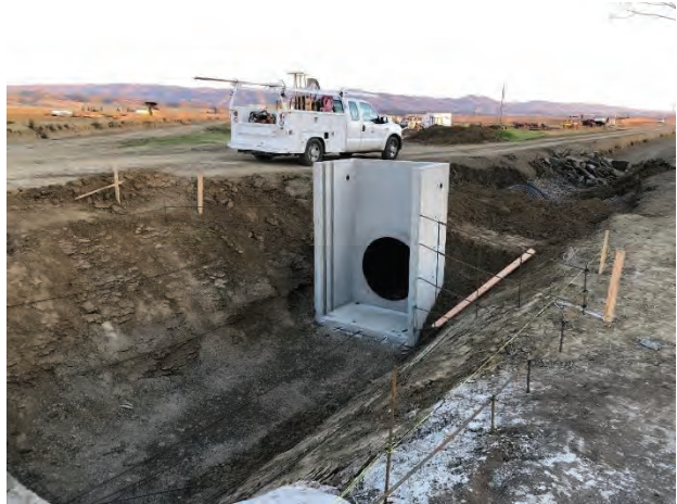
Fig. 3: Installation of Precast Heading Structure
