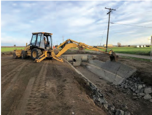
Fig. 2: Demolition of Existing Canal Heading
