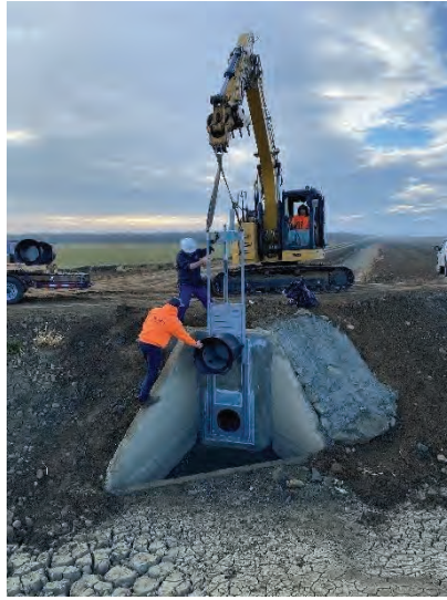
Fig. 9: Installation of PikoMeter
