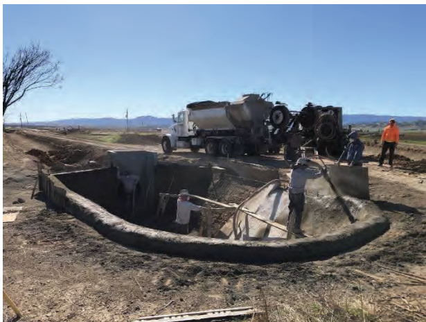
Fig. 4: Installation of Gunite for Stilling Pool
