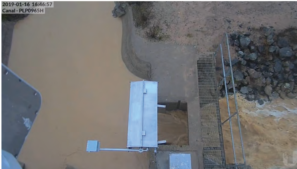
Fig. 14: SCADA Gate Surveillance of Storm Runoff Event
