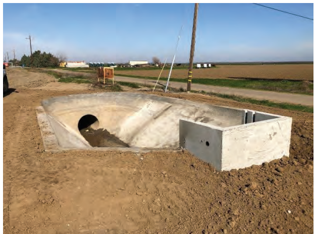
Fig. 5: Completed Civil Construction
