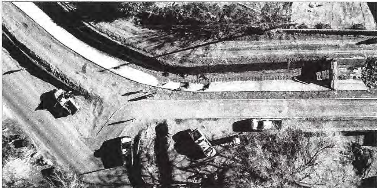
Figure 7. Ongoing Concrete Lining and Trail Construction at Montoya Main Lateral
