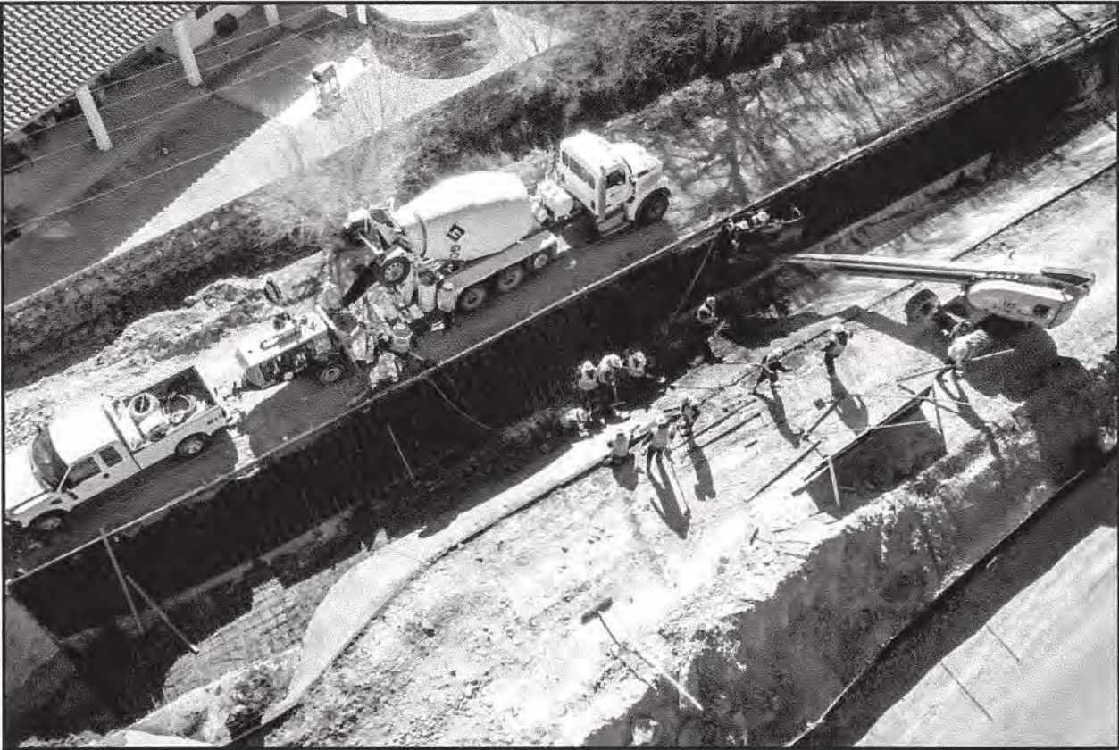
Figure 3. Cured Shotcrete and Liner and Steel Rebar Framework Ready for Shotcrete
