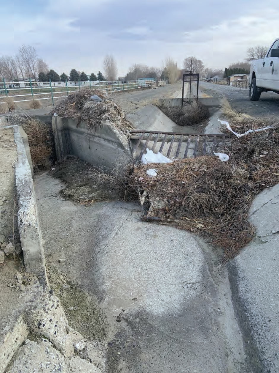
Lateral #1 Sands Wasteway
