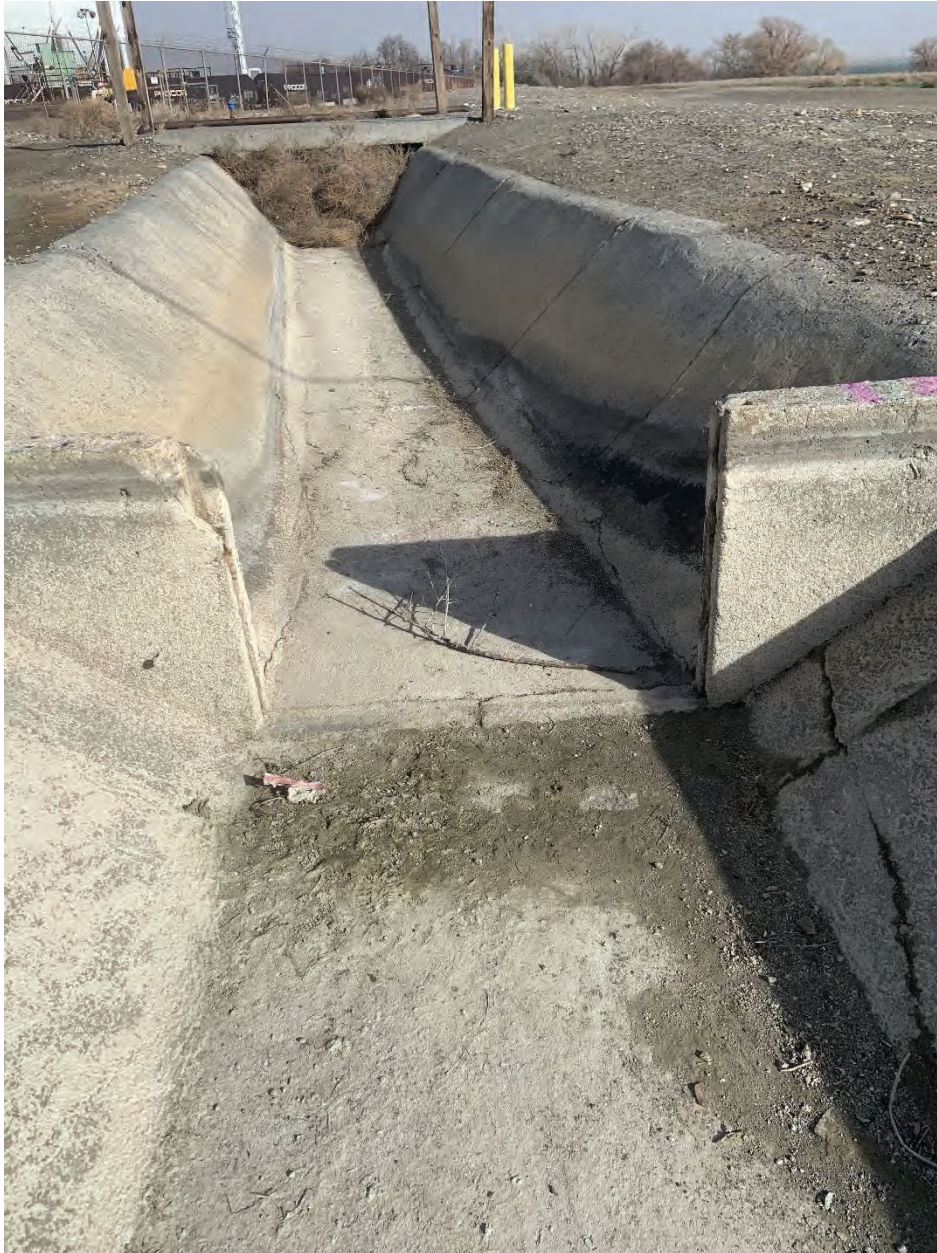
End of Lateral #2 Check
