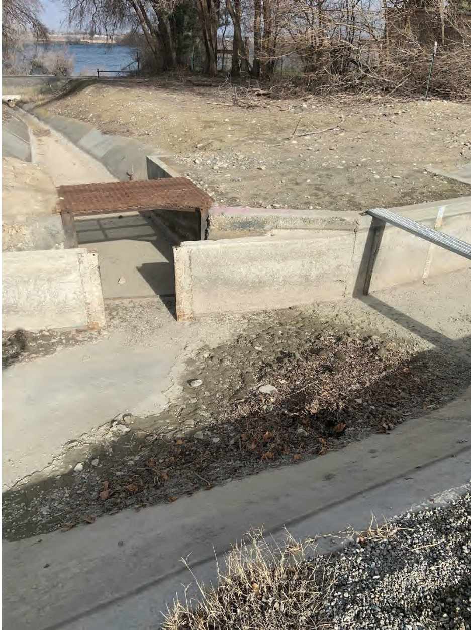
Lateral #2 Cox Wasteway
