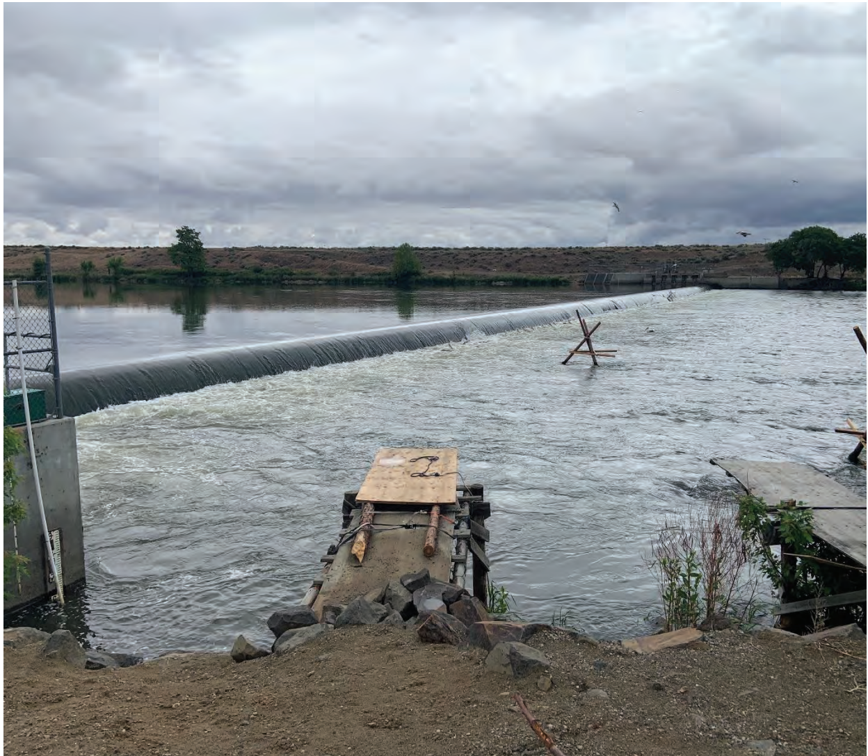
A View of Wanawish Dam
