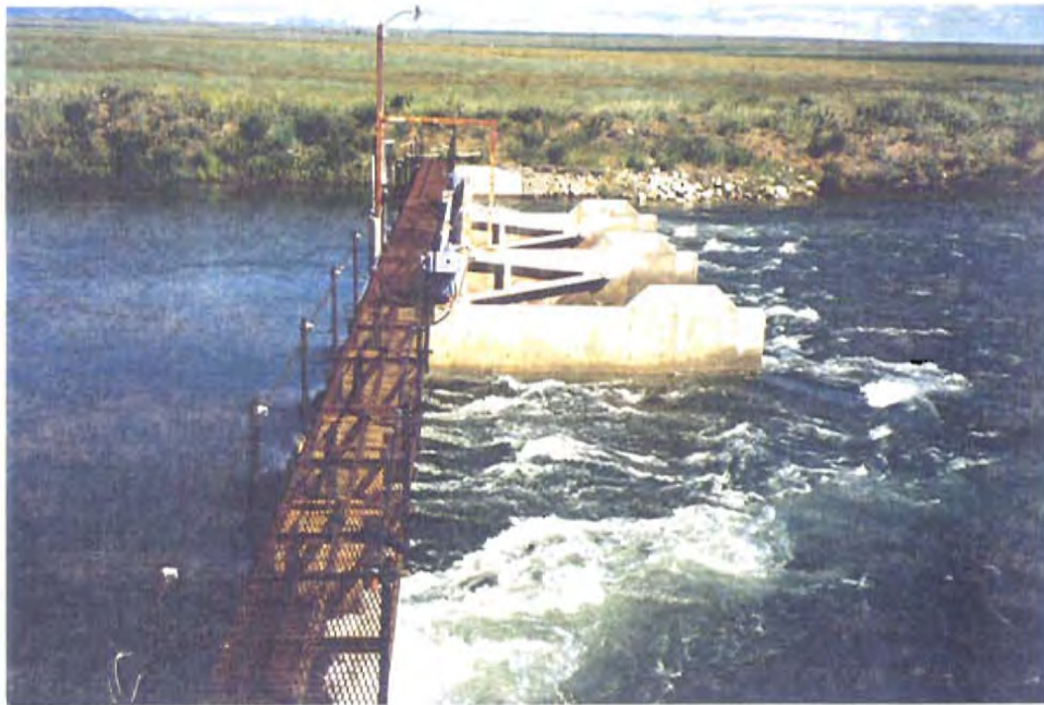
Photo 1 - SRS-71 Check (check #1)
