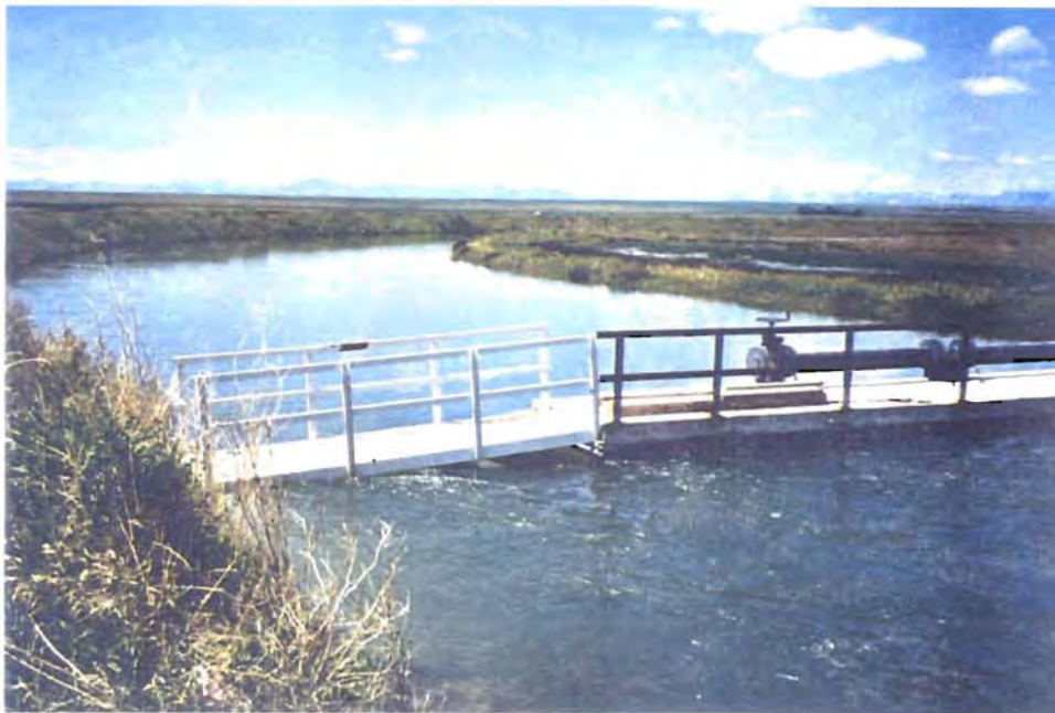
Photo 4 - SVC-35 Check (check #3)
