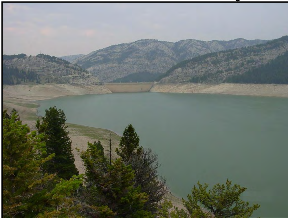
Photo 2. Gibson Dam and Reservoir near the end of the irrigation season.
