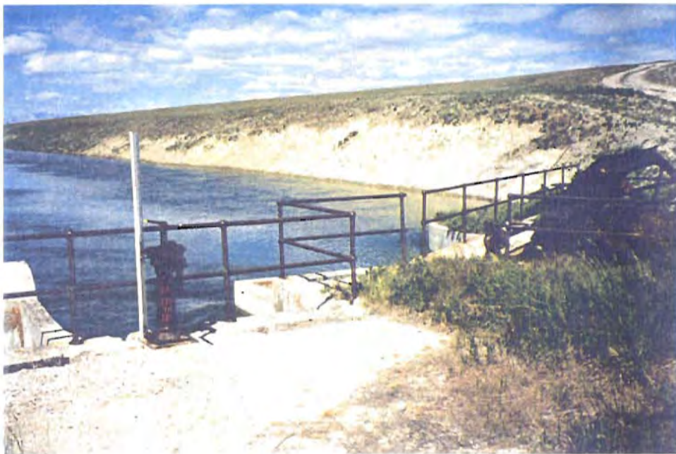
Photo 2 - SVC Headgate (check #2)
