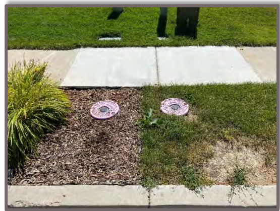
Photo 2 – Individually metered connections in RWCD's service area.
