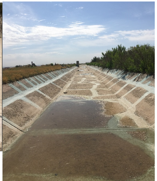
Photo 2: Main canal deterioration as shown in a Google Earth image. Note: 5 degraded areas over 300ft.
