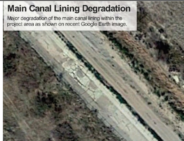
Photo 1: Existing condition of main canal within project area
