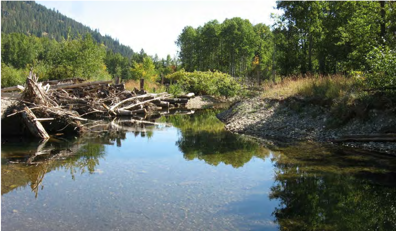
Figure 4. Example of inlet jam. Installed by Inter-Fluve 2013, photo taken in 2016 (Inter-Fluve).
