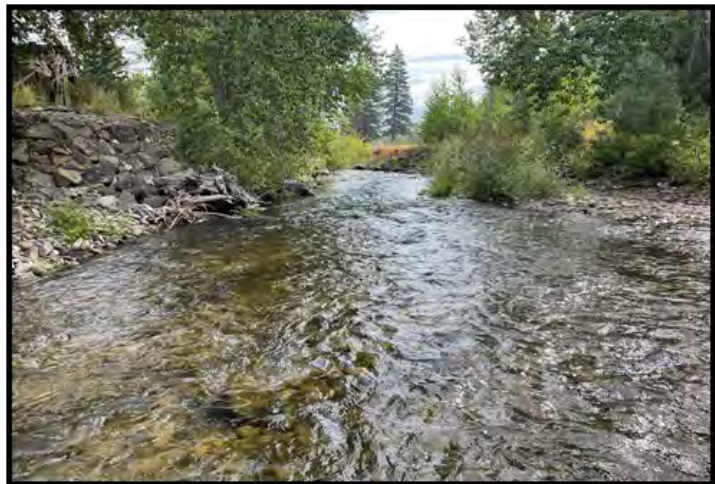
Figure 4. Image depicting armored banks of Warm Springs Creek, adjacent to the Warm Springs Preserve.
