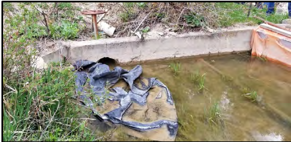
Figure 6. The project will upgrade the diversion infrastructure, including the head gate, flow measuring device, and fish screen.
