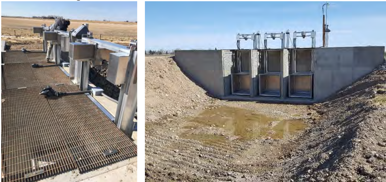
Figure 2. Phase I: Smart Check on GM100 constructed by GID 2020-21 funded in part by WaterSMART
