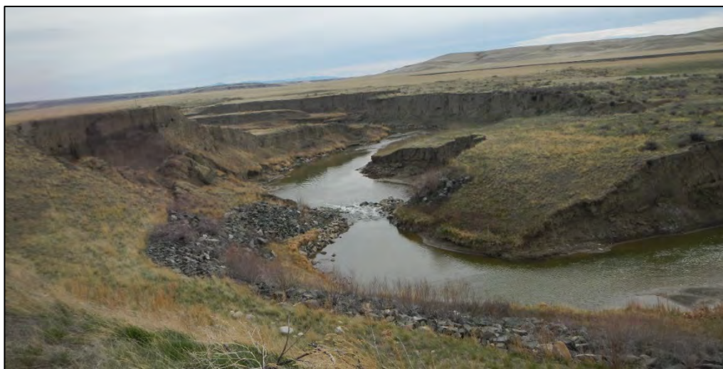
Photo 1, April 29, 2021. View downstream showing Muddy Creek drop structure within incised channel.
