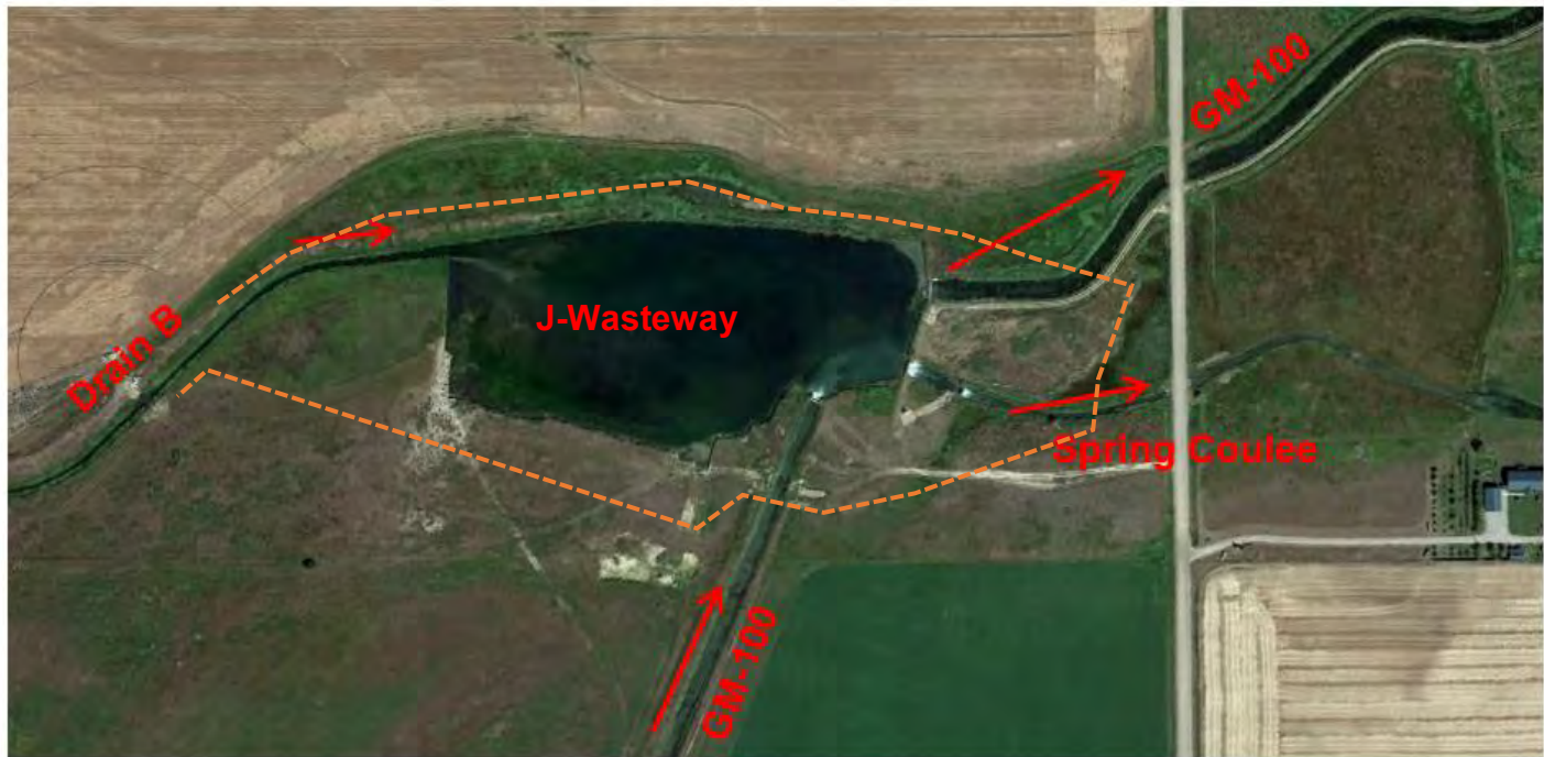
Figure 3. J-Wasteway re-regulation facility including inflows and outflows. Muddy Creek is located to the east outside the frame and receives water from Spring Coulee. The orange dashed lines indicate the berm alignment to enlarge the re-regulation capacity.
