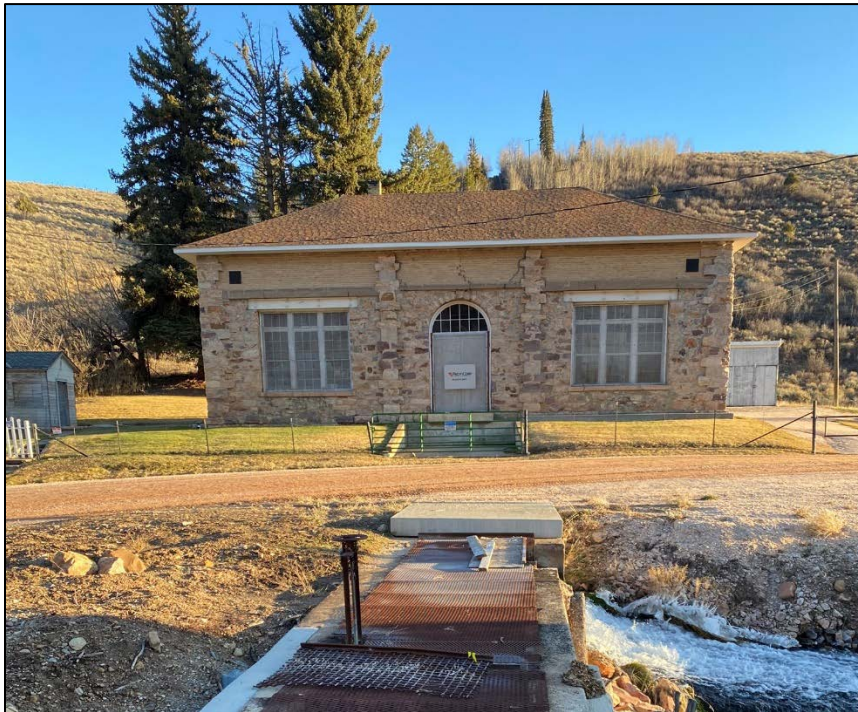
Figure 3. Photo of the Paris Hydropower plant as taken from the tailrace on November 17, 2021. The tailrace is piped under the graveled Paris Canyon Road. The buildings, pipe under the road, and some tailrace features will be removed with decommissioning.
