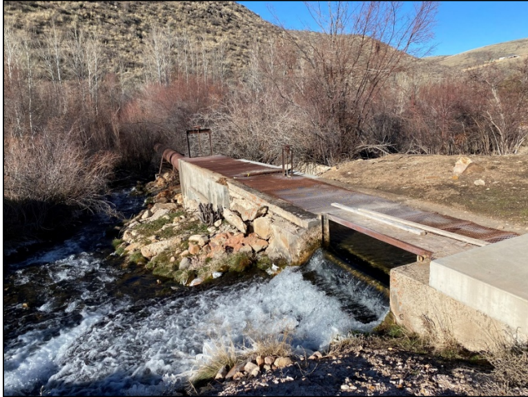
Figure 4. Photo of the Paris Hydropower plant tailrace taken on November 17, 2021. As shown, all power plant flows are being returned to the creek after the irrigation season. The portion of the concrete flume with the headgates will likely remain with the new irrigation pipeline entering at this point to send water to both canals.
