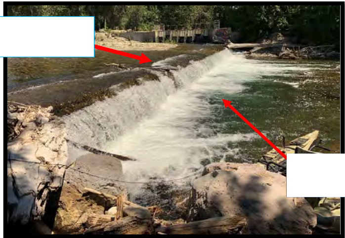
Photo 1 Diversion 45 Existing Condition
