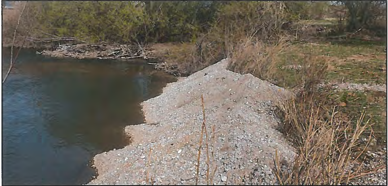
Photo 12. Unprotected gravel dredge material on river bend, sample of gravel accumulation areas
