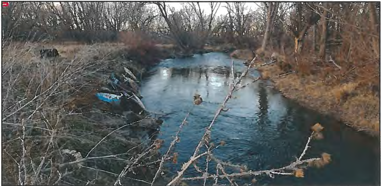
Photo 8: Looking at multiple cars downstream of the diversion structure
