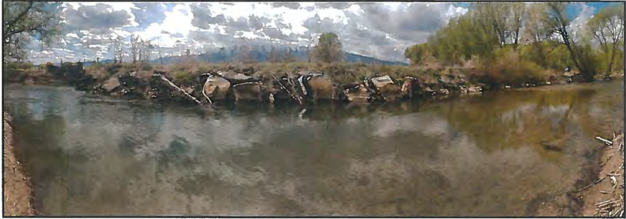
Photo 9: Cars armoring the banks, area of silt accumulation from upstream bank erosion
