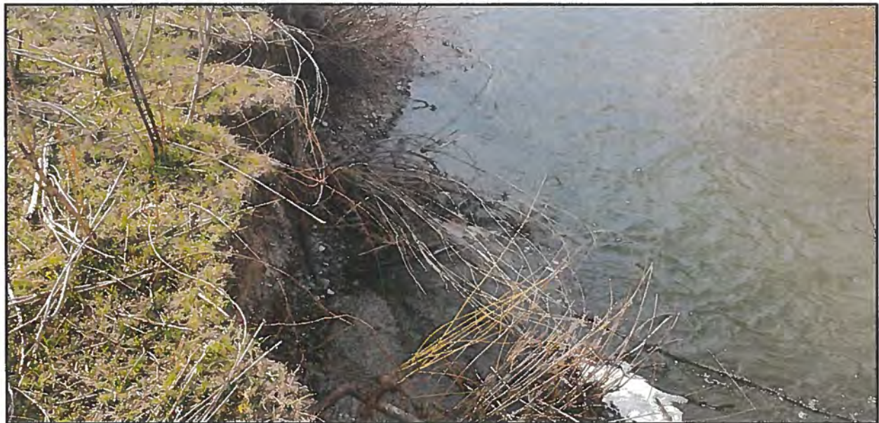
Photo 14. Vertical bank resulting from devegetation and over grazing
