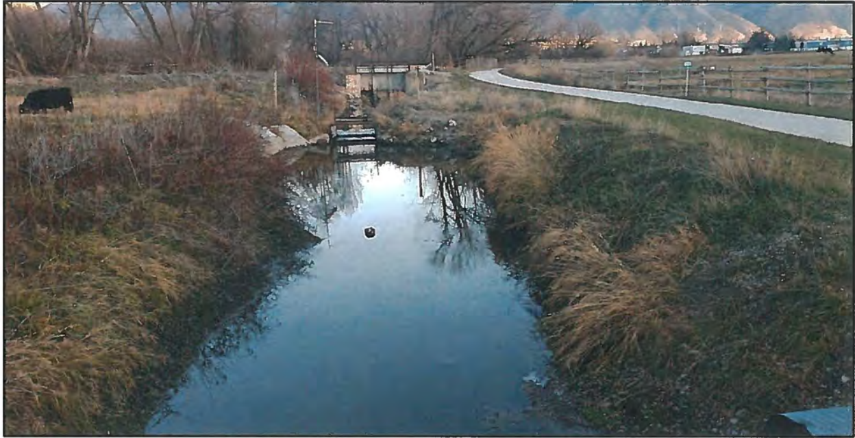
Photo 16. Existing Canal below existing measurement flume
