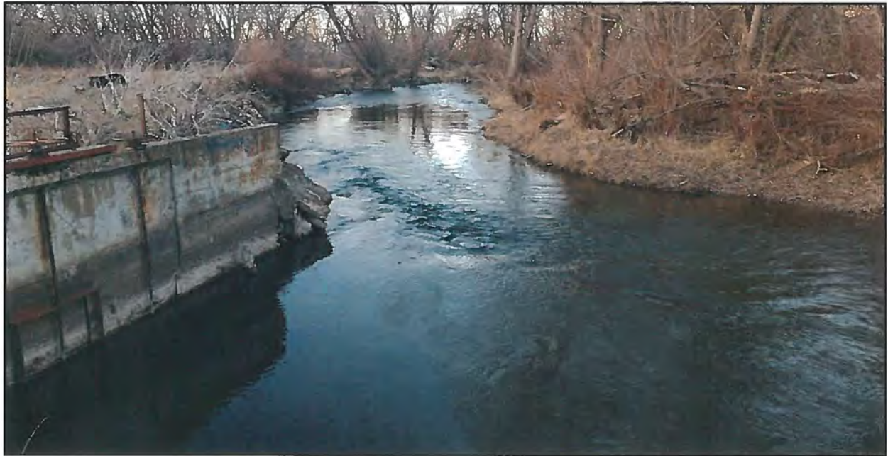
Photo 1: Existing diversion structure looking downstream
