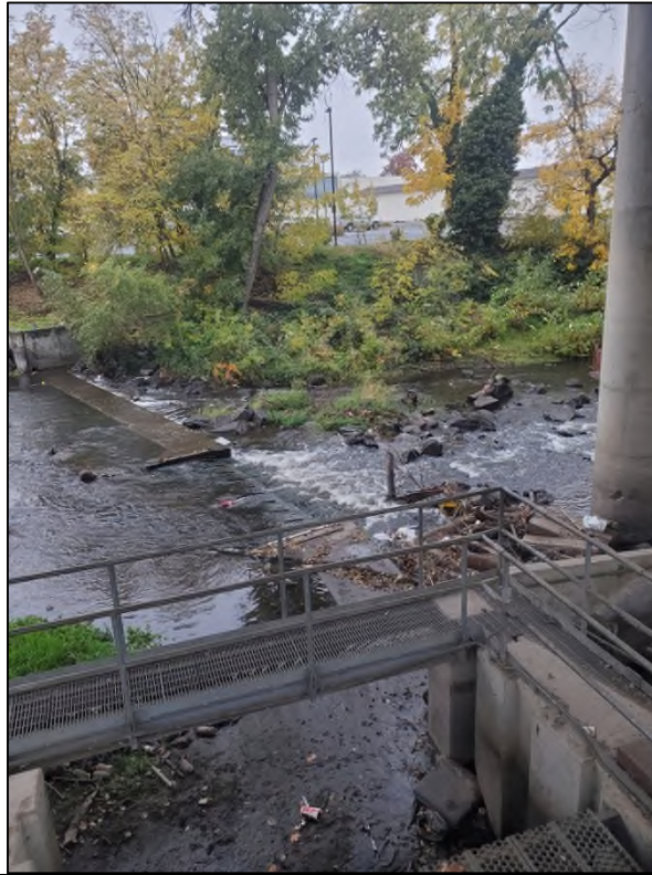
Photo 7 (September, 2021): Structure #4 (RRVID intake) standing on river right looking downstream.
