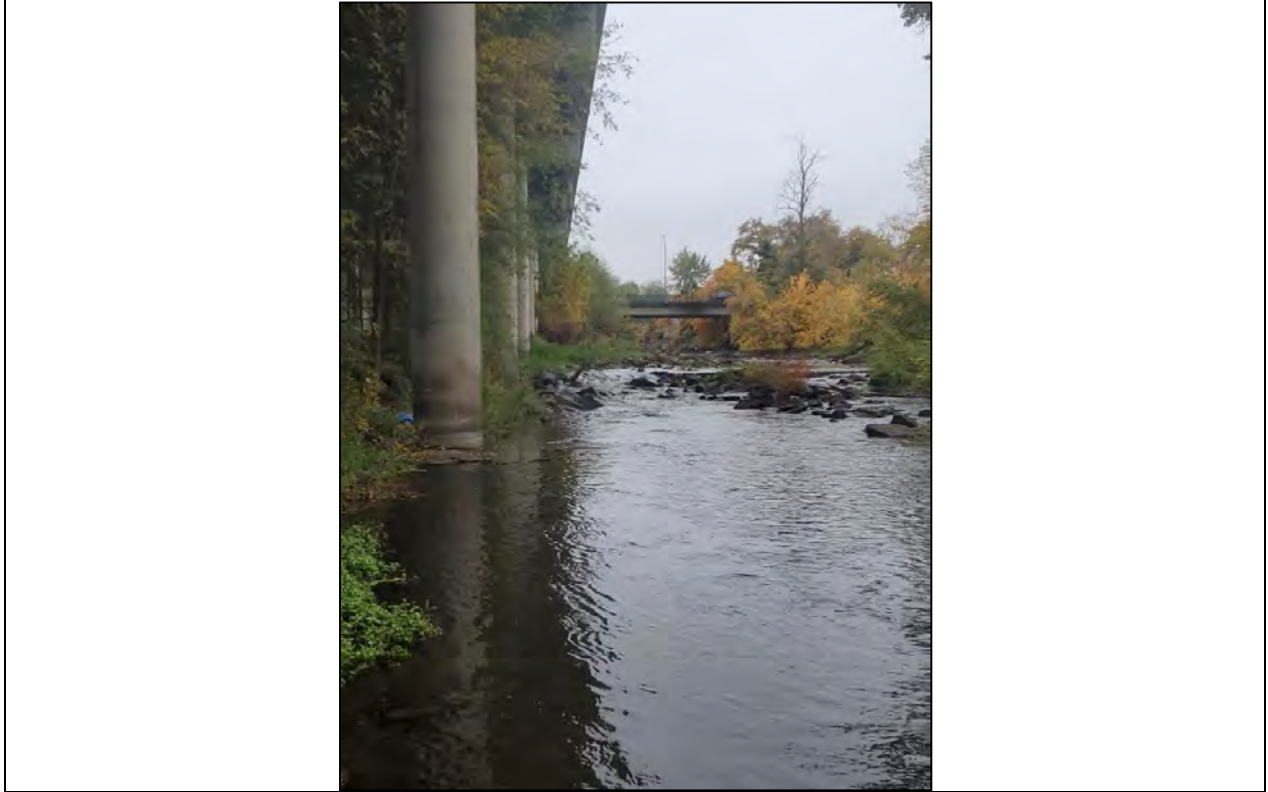
Photo 9 (September, 2021): Structure #4 (RRVID intake) standing downstream looking upstream.
