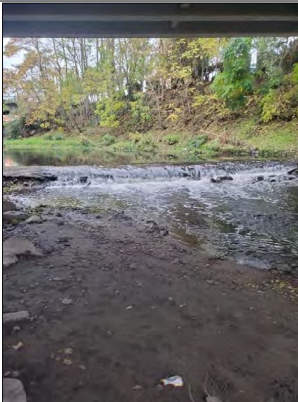
Photo 6 (September, 2021): Structure #3 (sewer line) standing downstream looking upstream.
