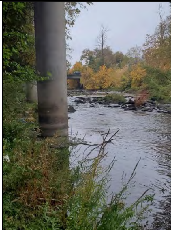
Photo 8 (September, 2021): Structure #4 (RRVID intake) standing downstream looking upstream.
