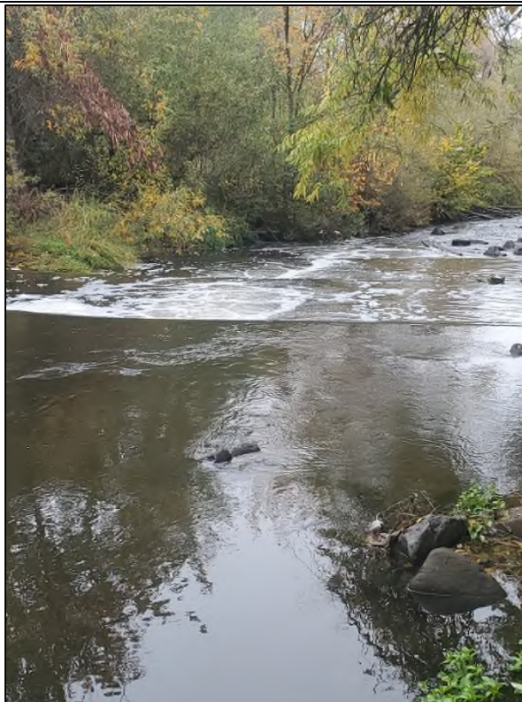
Photo 2 (September, 2021): Structure #1 (weirs) standing upstream looking downstream.
