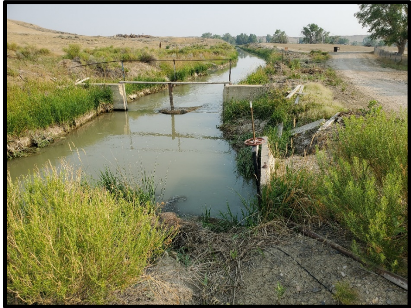
Photo 2 Existing Condition of the D52 Lateral
