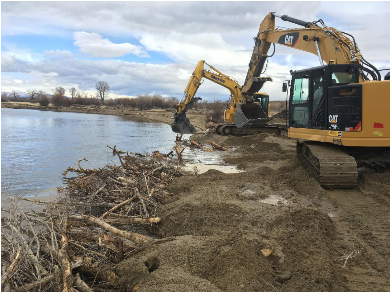
Photo 2 – Toe wood provides bank protection and cover for fish until vegetation establishes.
