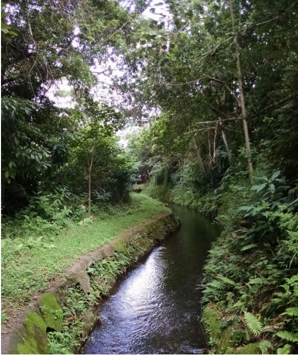
13 A network of ditches tap streams draining from the fence units to supply municipal and agricultural needs.
